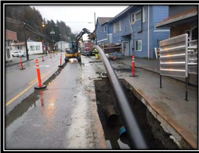
Using HDPE pipe to Slipline a sewer force main in Ketchikan.
