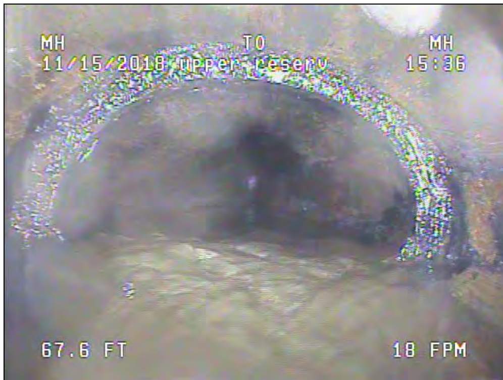
Collapsed joint in the 8-inch woodstave conduit, 2018 inspection.
