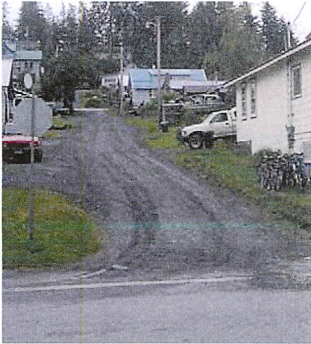
“Weber Street – Example of a Wrangell street that needs paving”
