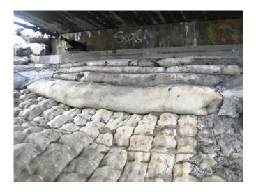
During the recent wind storm that Wrangell endured a few weeks ago, several completed pile wraps were damaged by the summer float which was ripped away from its secured location. NUC has been asked to replace the damaged wraps, and will be compensated on a time and materials basis through a subsequent change order. NUC is still on schedule for project completion by mid-October 2012.
