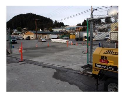
• The above picture shows the approach way into the yard that was paved as part of this contract. This leveled out the road provided drainage solutions for both the City and the adjacent business and now that it is paved, eliminates a lot of the mud that was brought into the yard when vehicles would drive through the dirt road and mud puddles.
