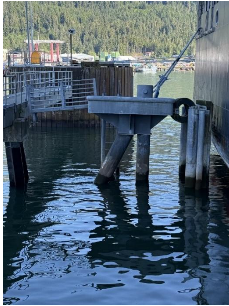
Figure 8 City Dock Mooring Dolphin
