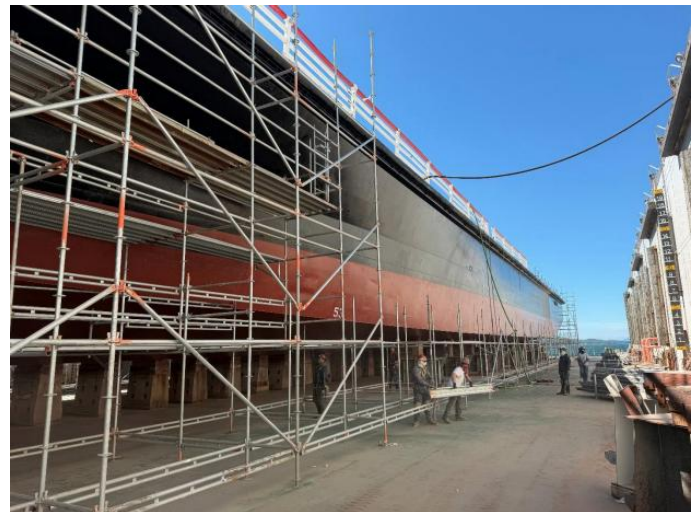
Figure 7 American Empress Under Construction
