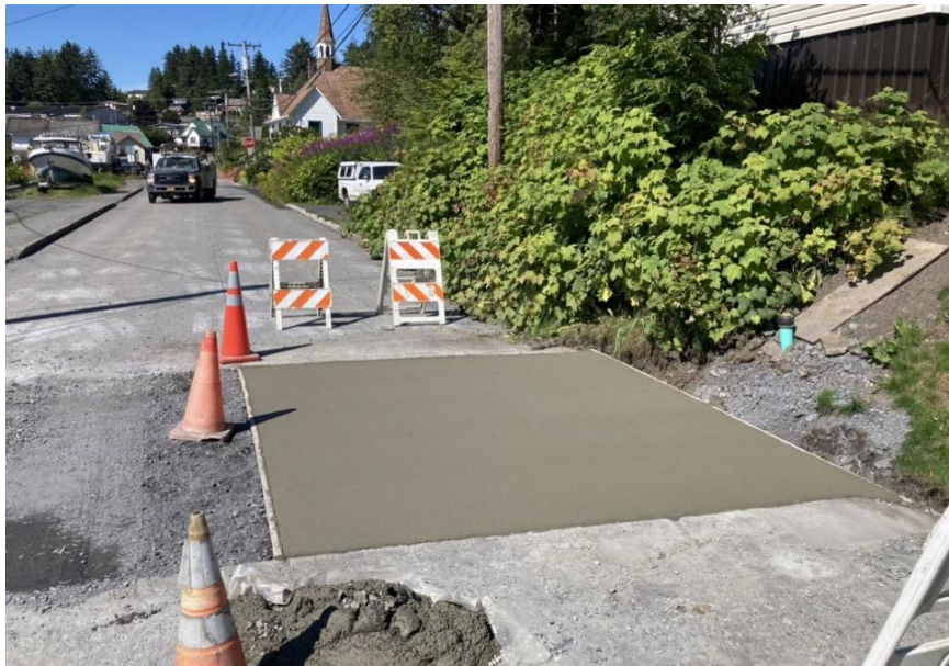
Figure 11 Lower Church Street Concrete Patching
