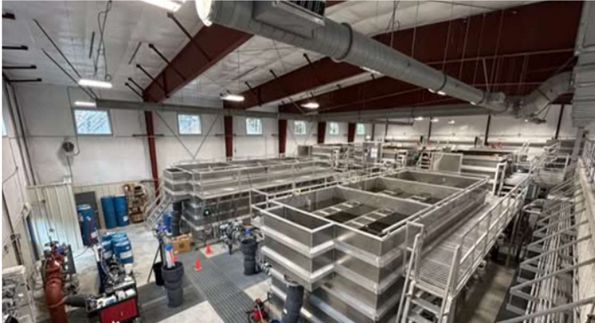
Inside the new Wrangell Water Treatment Plant emphasizing the DAF train units.
