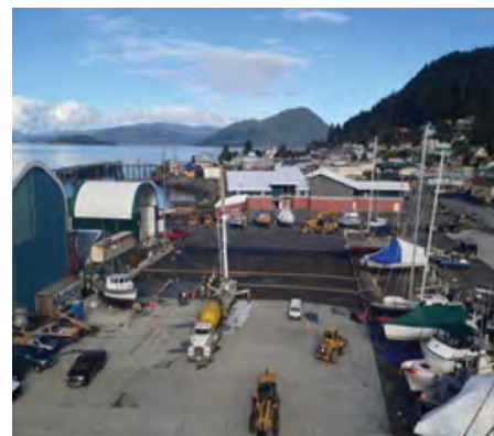
Wrangell Marine Center (PND Engineers)
