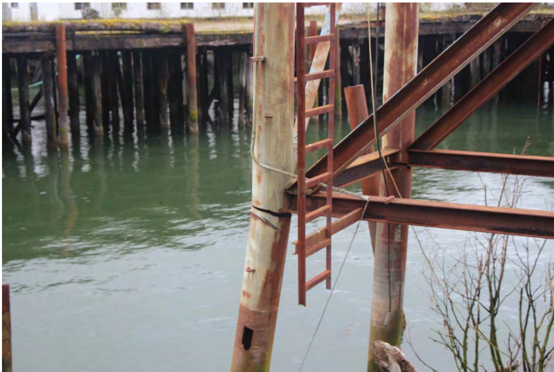
Photo 5 – Failed Column at Shore-side Conveyor Tower
