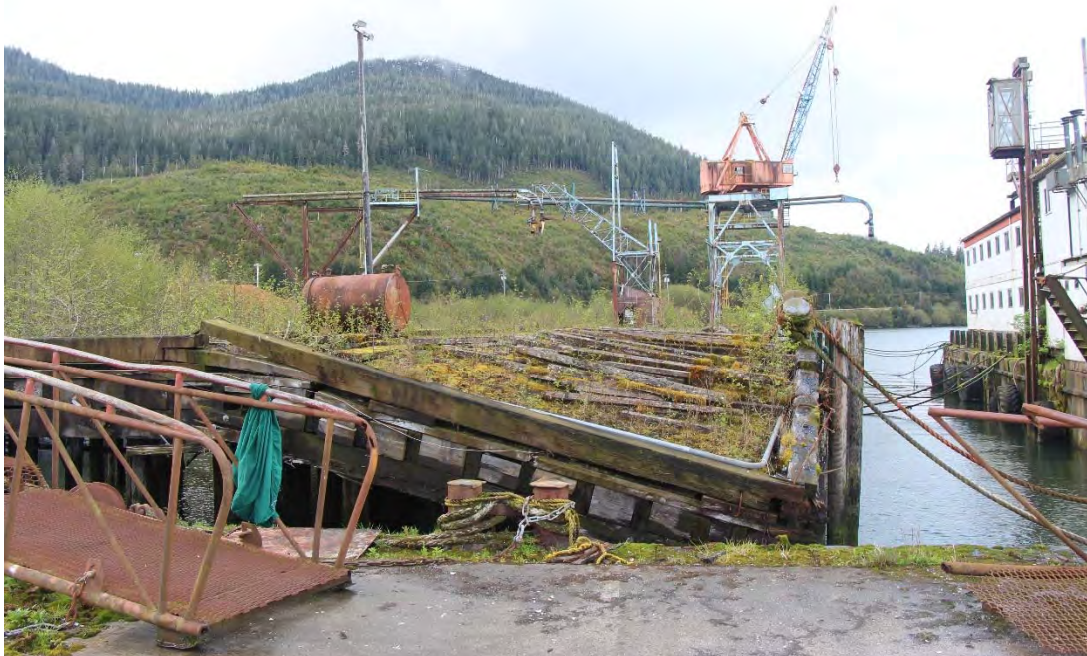
Photo 4 – Damage at North End of Timber Pier
