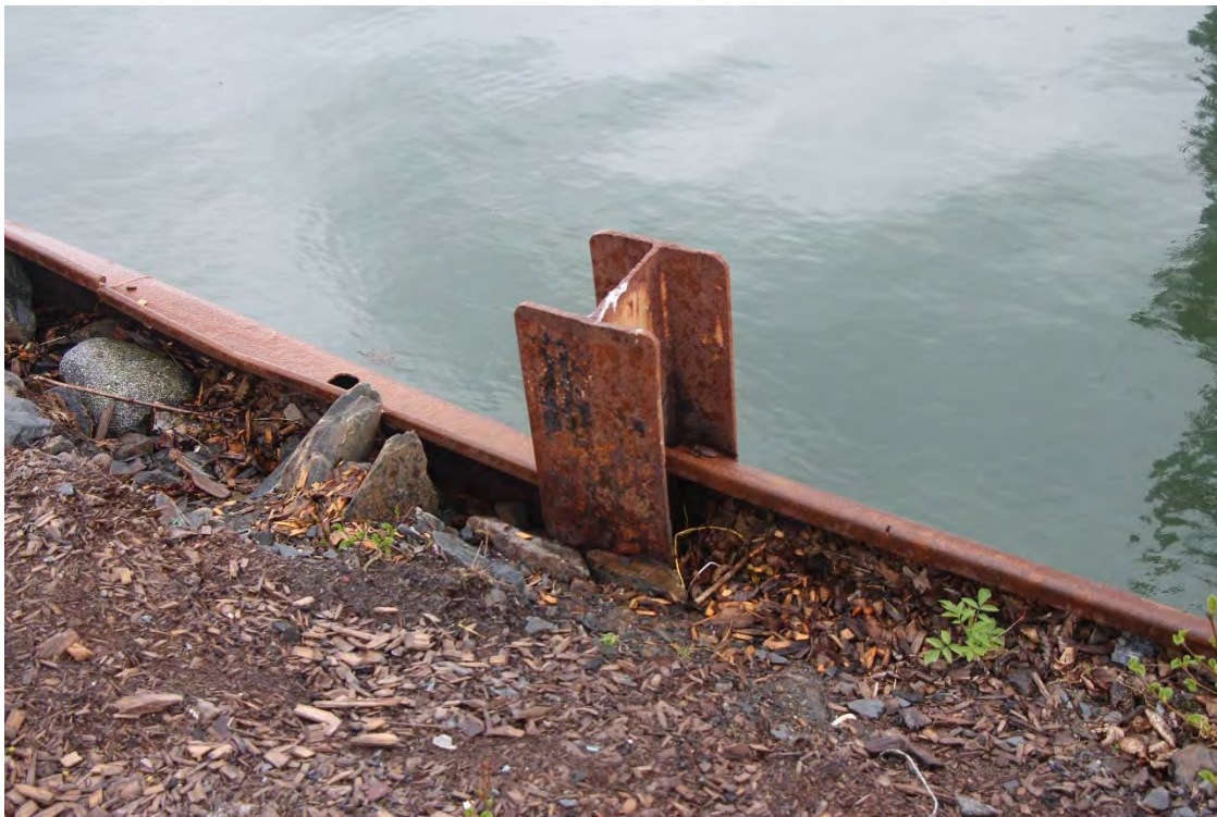
Photo 7 – H-Pile at Railroad Car Bulkhead
