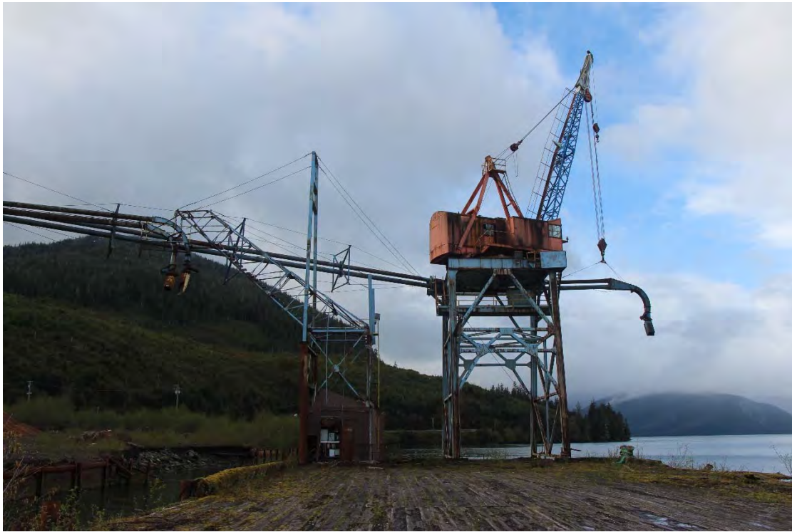
Photo 5 –Tower Crane and Conveyor Support
