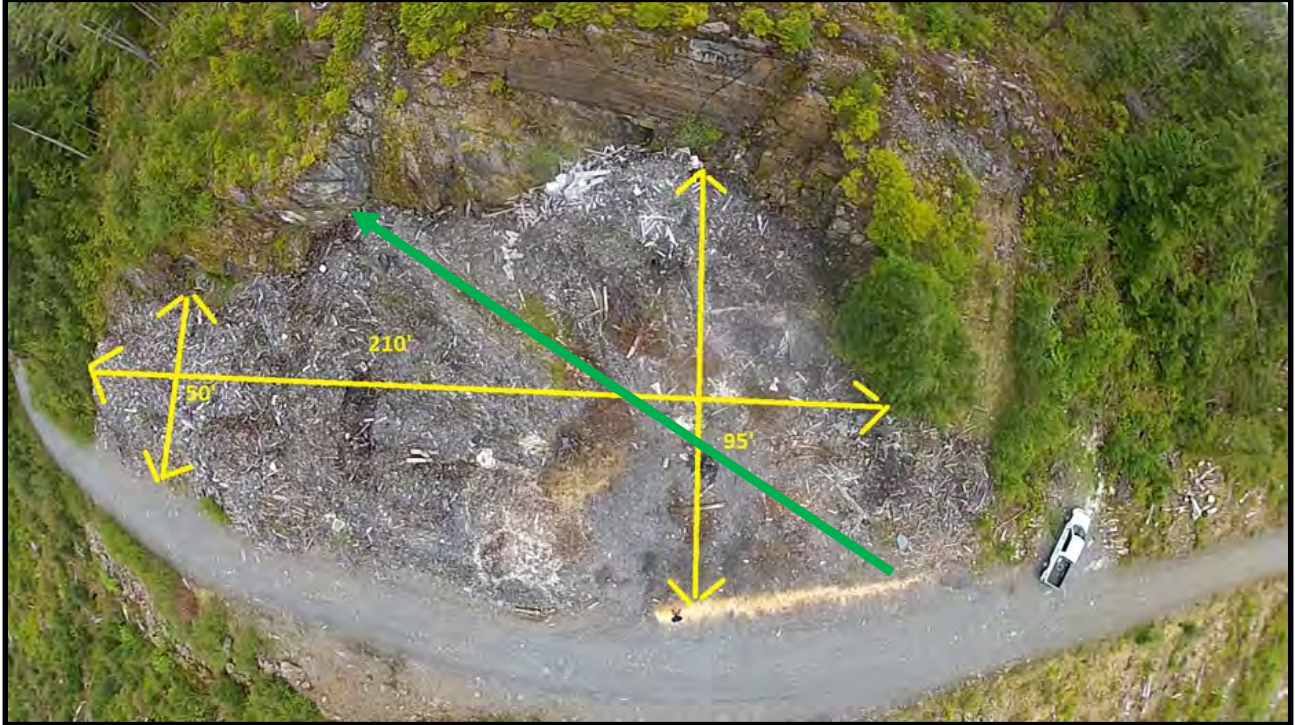
Photo 1: Aerial photo showing Spur Road Rock pit as potential monofill location for treated soil from Wrangell Junkyard. Rock pit is on the ocean side of Spur Road. Fisheye lens is providing some distortion, but overall site layout is basically as shown.
