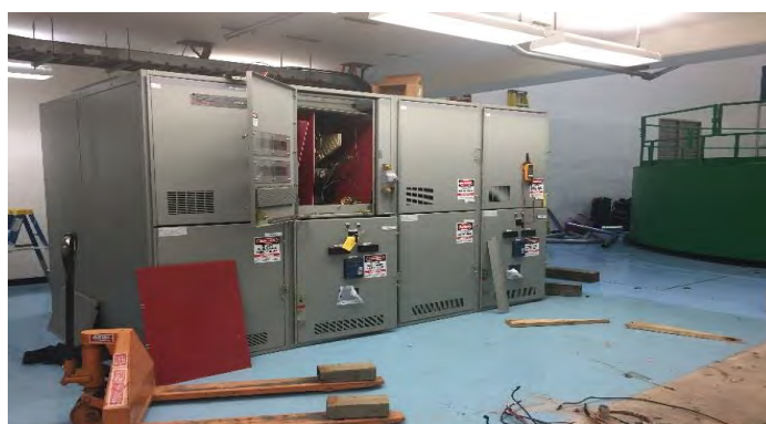
Unit 1 New Switchgear Cabin Installed
