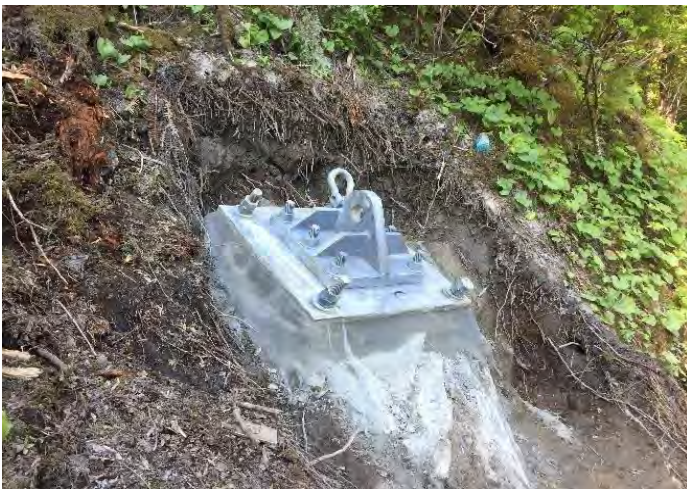
New Debris Boom Shore Anchor (Complete)
