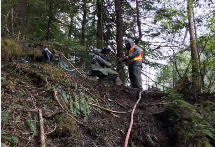
Hand Drilling Shore Anchors
