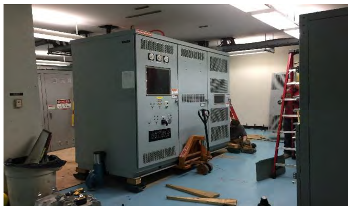
Removing Unit 1 Exciter Cabinet
