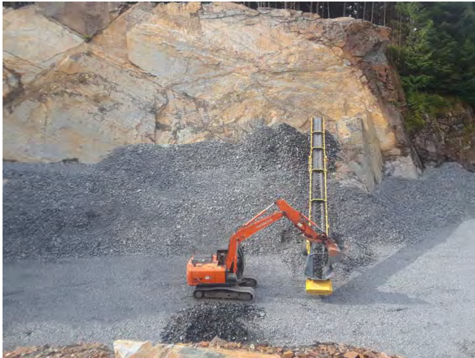
Photo 1: Monofill Site, using conveyor to place rock for Chimney Drain
