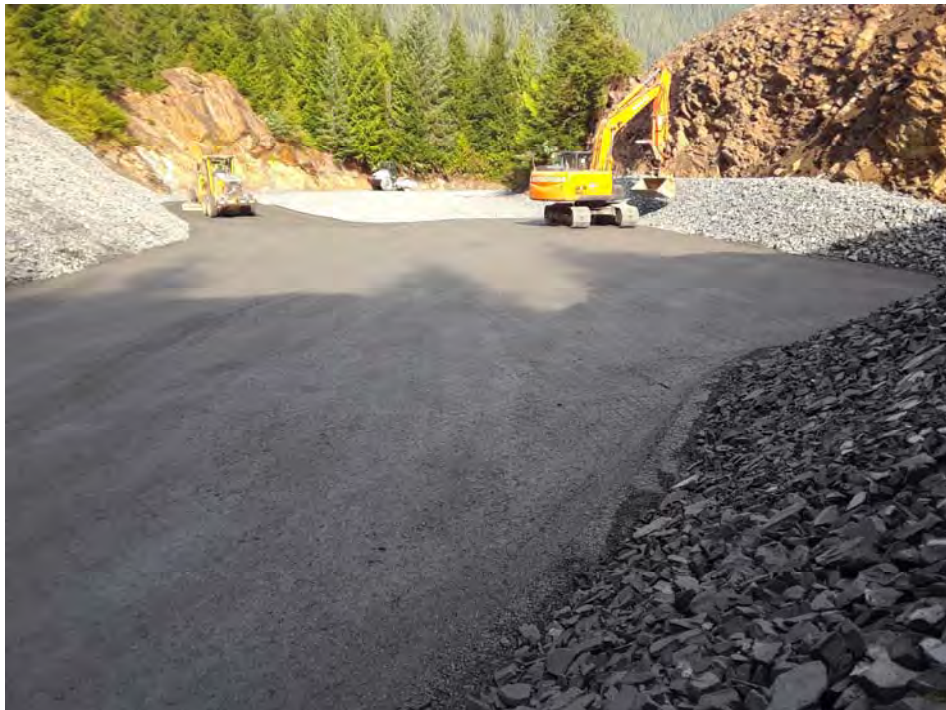
Photo 2: Placing skim layer of D1 over Base Drain, September 21, 2017
