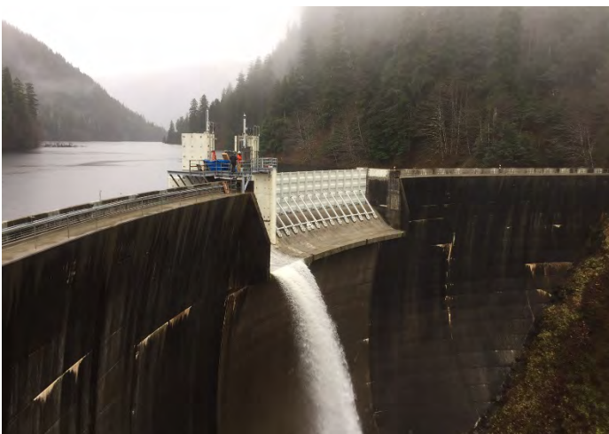
Testing the new vertical gate system at Swan Lake
