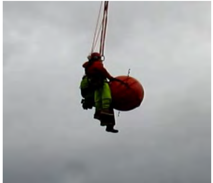
Over 100 Tyee transmission line marker balls were updated with larger, higher visibility replacements. The old original balls were faded, and some had slipped in position. Marker balls are attached to overhead transmission lines to make them more visible in areas frequented by aircraft. This challenging removal and installation job required a specialty crew, with two linemen suspended on a longline from a helicopter!
