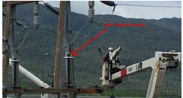
Replacement of 98kV Maximum Continuous Operating Voltage (MCOV) Surge Arresters located in the Bailey Substation.
