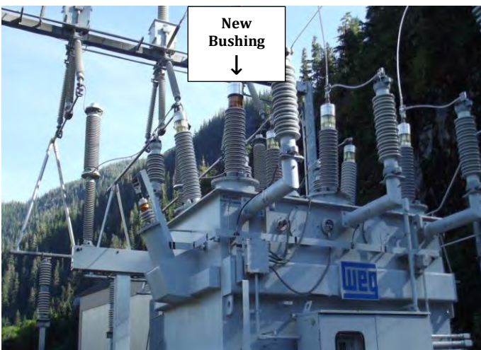
A damaged transformer bushing was replaced in Tyee Switchyard.
