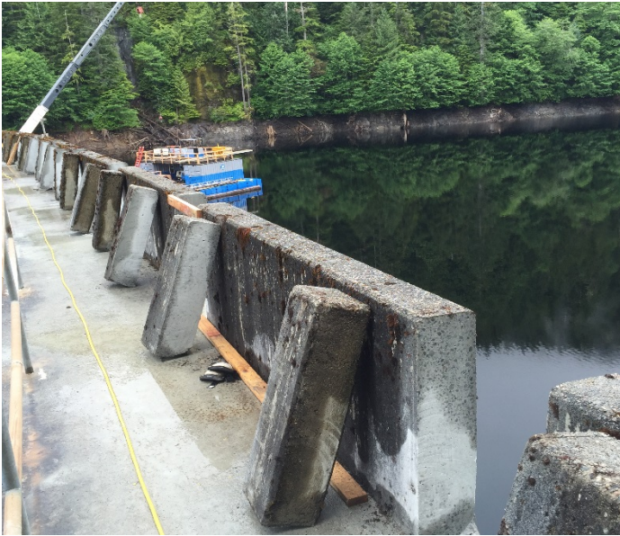
Parapet Wall Concrete Excavation
