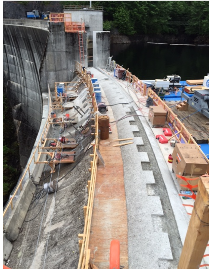
Spillway Concrete Excavation
