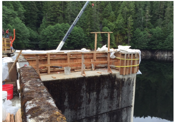
South Pier Height Increase
