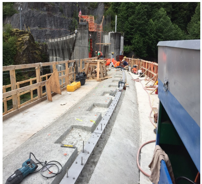
Flashboard Sill Plate Leveling
