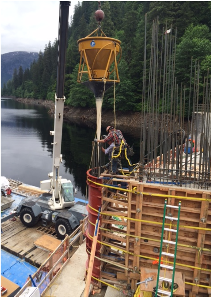
Middle Pier – Going Up!
