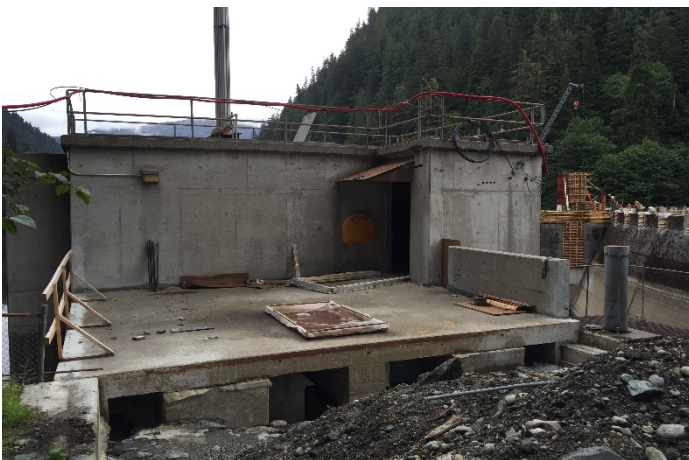
Intake Structure Excavation
