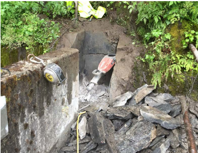
Left Dam Abutment - Parapet Wall Key
