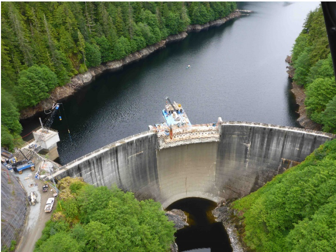
Swan Lake Dam – Construction Site
