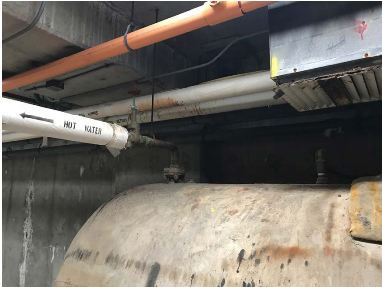
Existing Hot Water Tank – Plumbing Works
