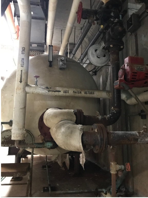
Existing Hot Water Tank – Plumbing Works
