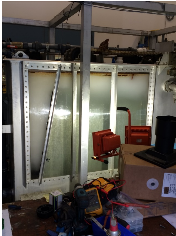
Figure 6 - Pilot Plant DAF Unit
