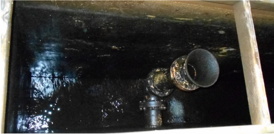
Figure 3 - Ozonated Water Connection
