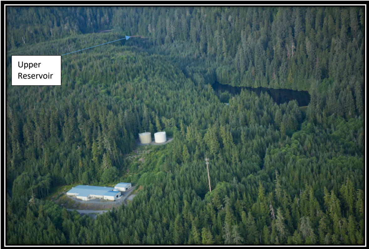
Water Treatment Facility
