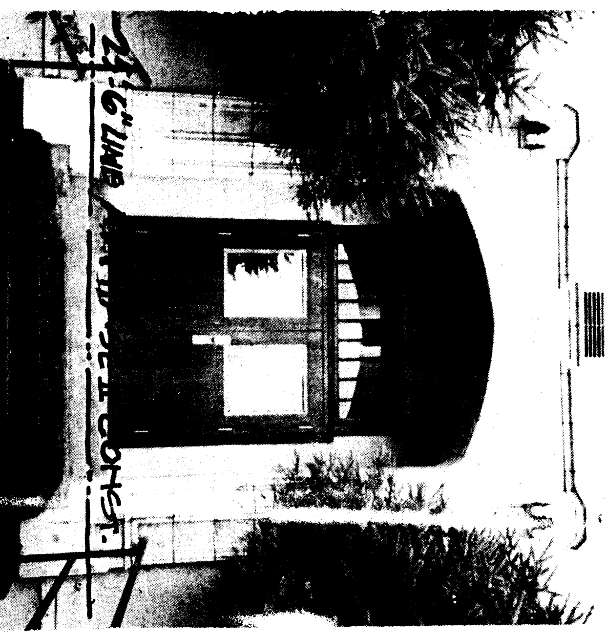
PHOTOGRAPH ELEVATIONS AT EXISTING TERRA COTTA ARCH TO BE REMOVED
