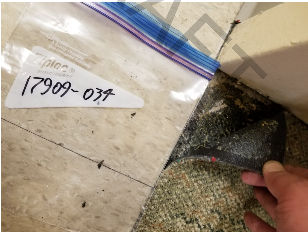
Photo 4: Black mastic beneath found beneath floor tiles and green carpet in the basement. (May 22, 2018)
