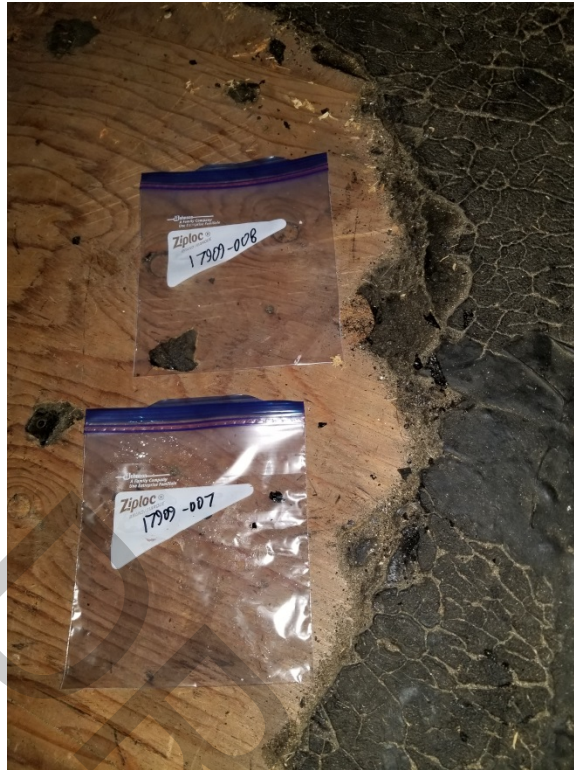
Photo 1: Roofing material of the original building roof is ACM. (May 22, 2018)
