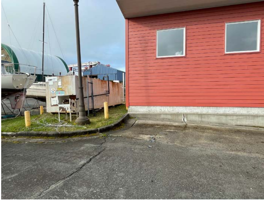
East Elevation Storage Building
