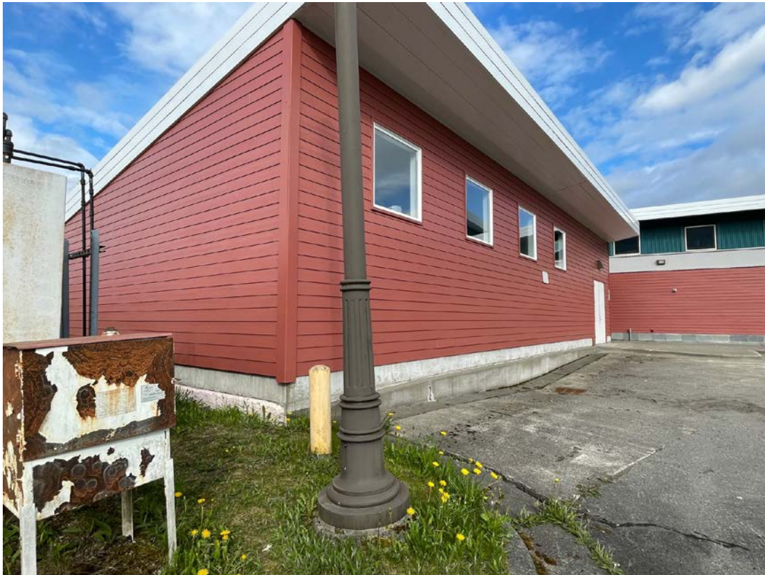
NOLAN CENTER STORAGE BUILDING SETTLEMENT REPAIR
