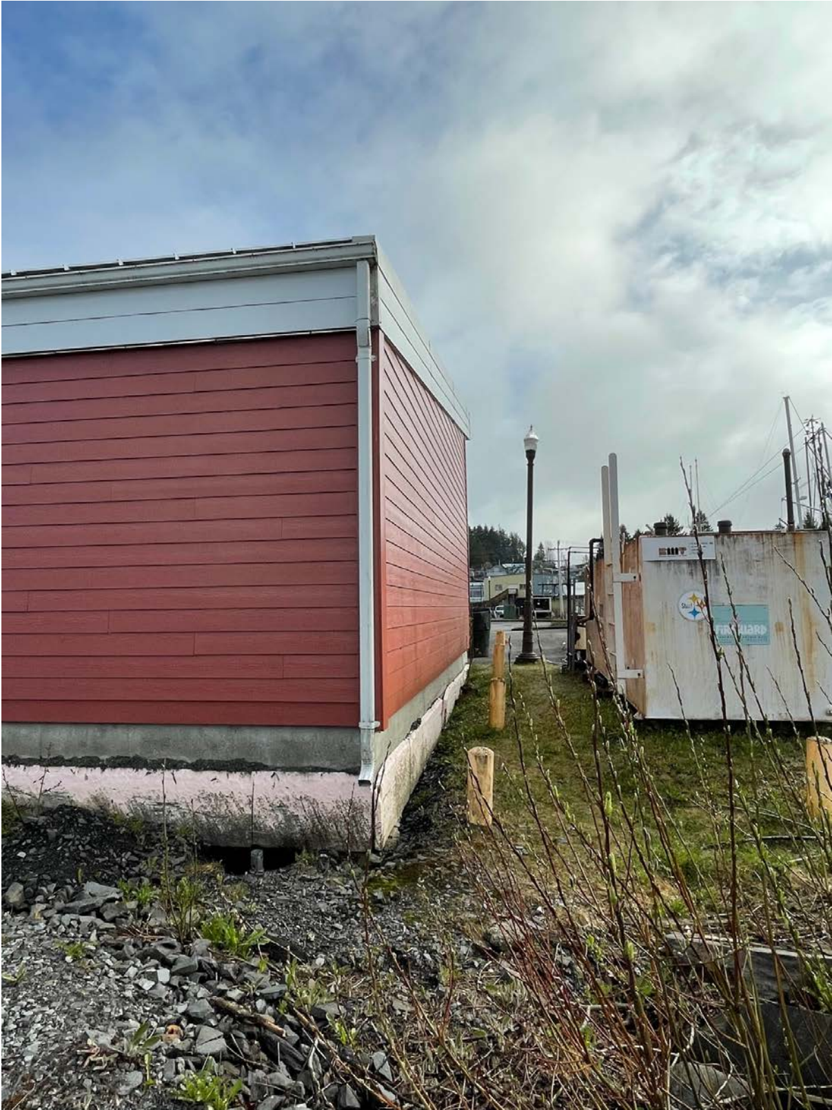
NOLAN CENTER STORAGE BUILDING SETTLEMENT REPAIR
