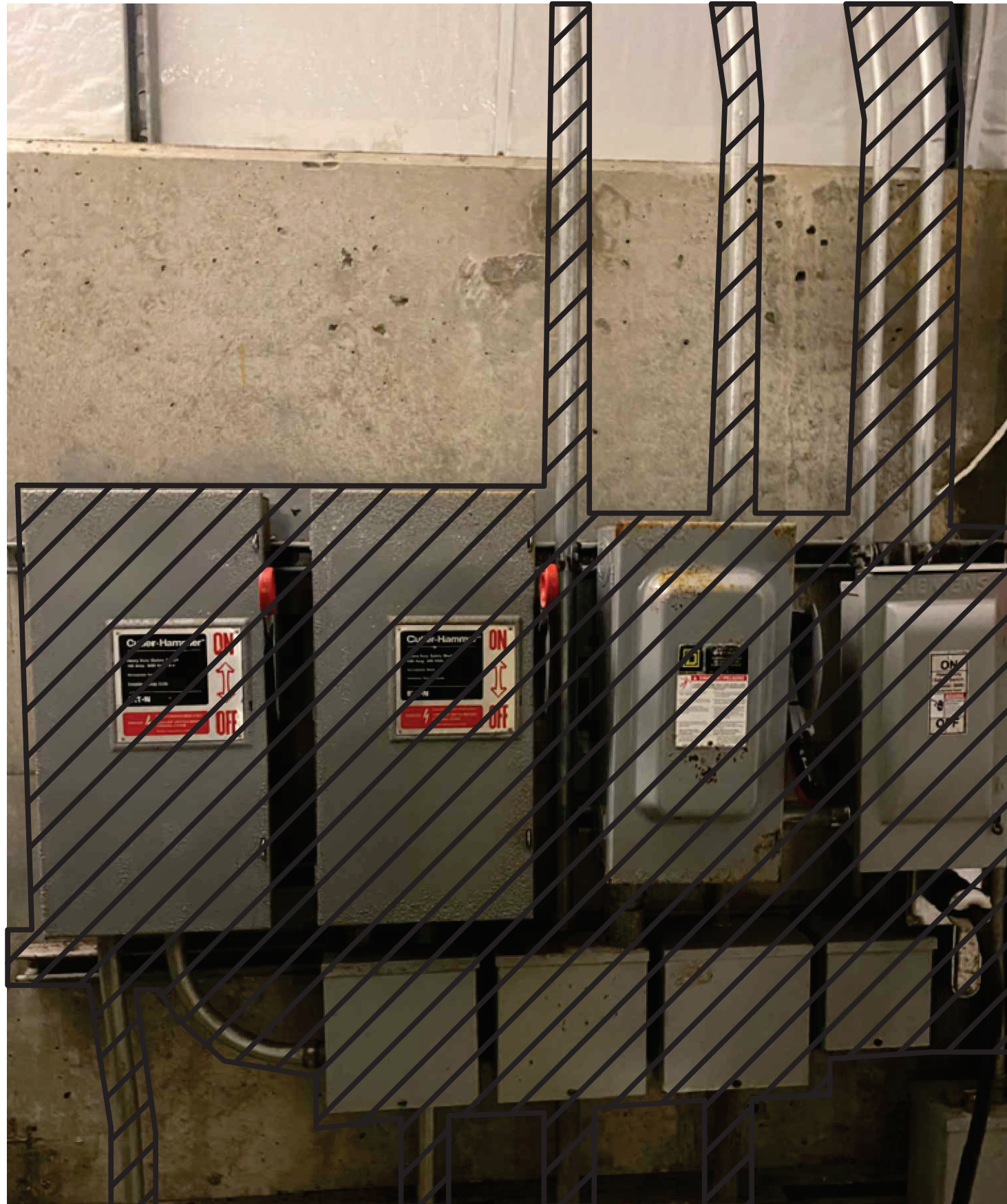
1 CLEARWELL BUILDING ELECTRICAL EQUIPMENT (DEMOLISH)
