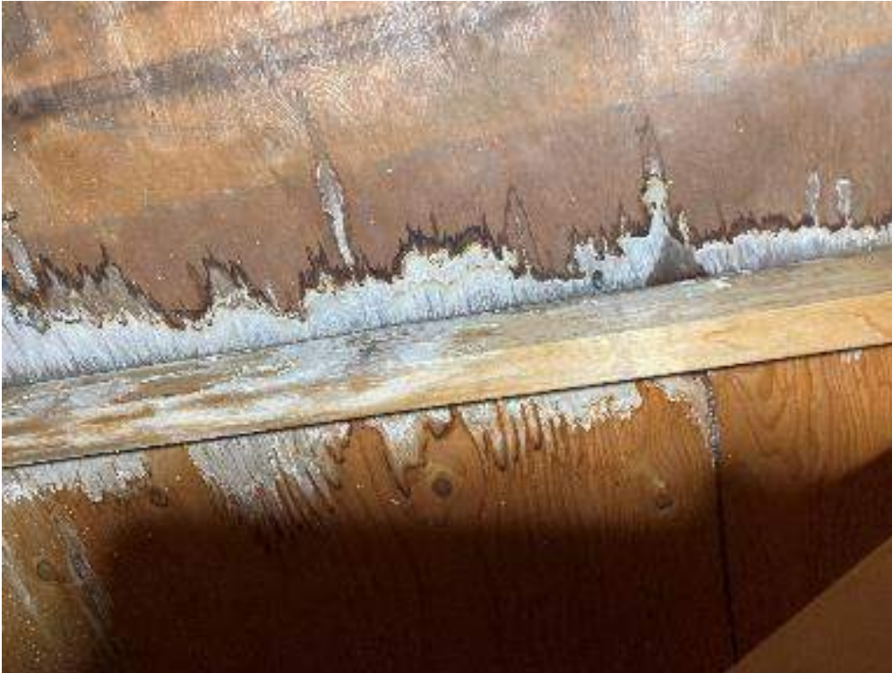
Water staining at roof sheathing
