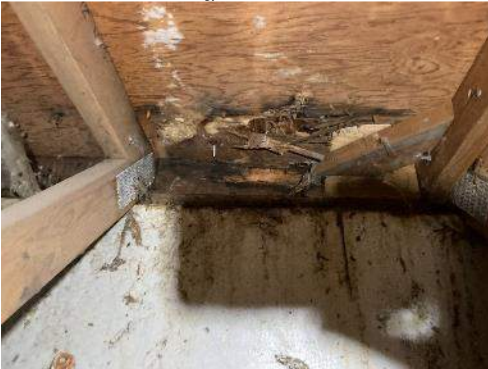
Rot at sheathing, blocking.
