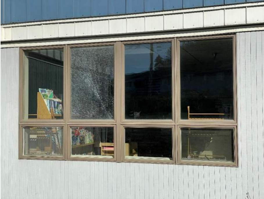
Broken glass in typical 4-modual unit, West elevation
