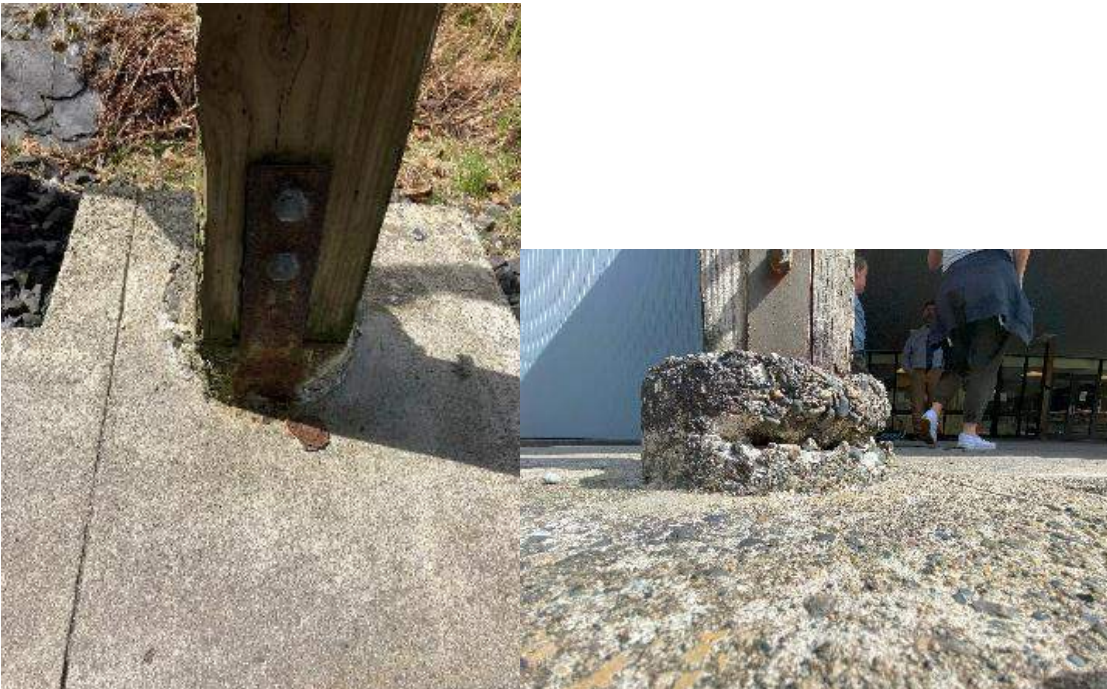
Deteriorated post bases
