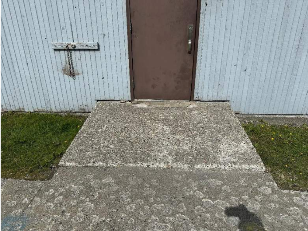
One of two concrete stoops recommended for replacement.
