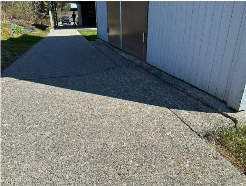
Differential settlement between sidewalk and foundations on west side of building
