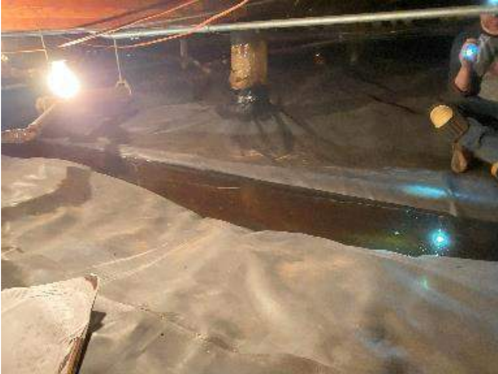
Water in Crawlspace (on top of Vapor Retarder)
