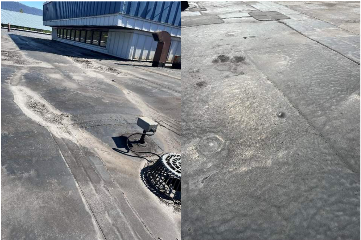
OSB “pillowing” at valley area, and debris under membrane
