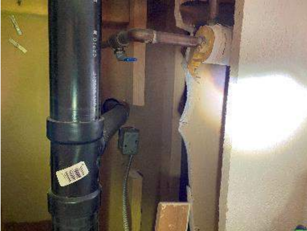
Cut structural studs.
