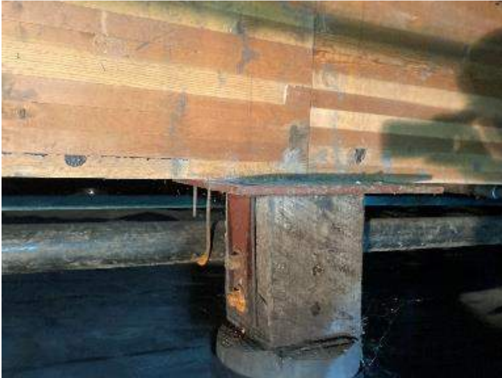
Missing connection plate.
