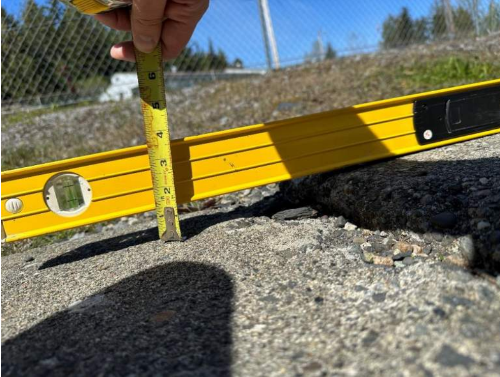
Abrupt elevation change (1.25") in sidewalk on west side of building
