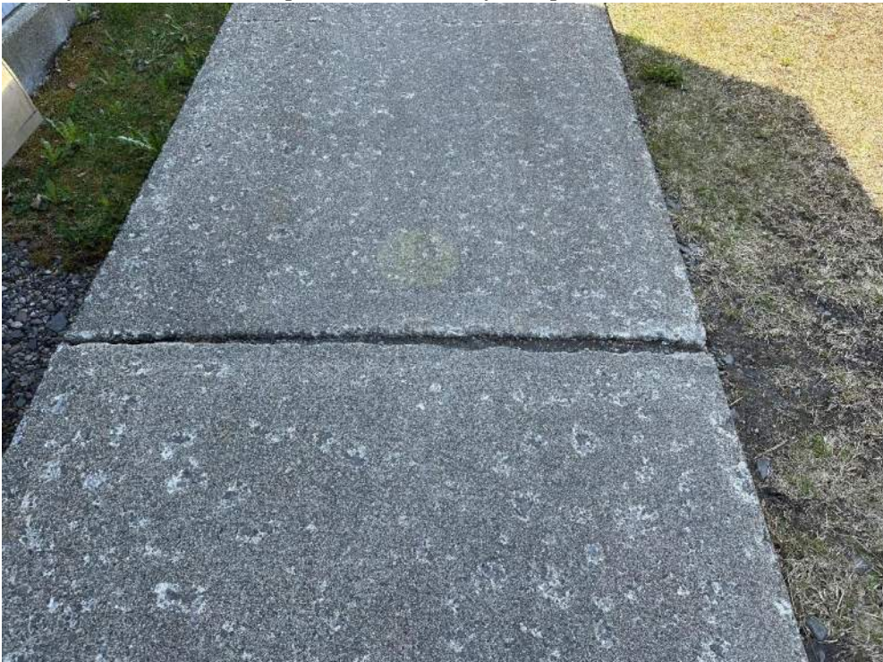
Large gap at joint in sidewalk on west side of building
