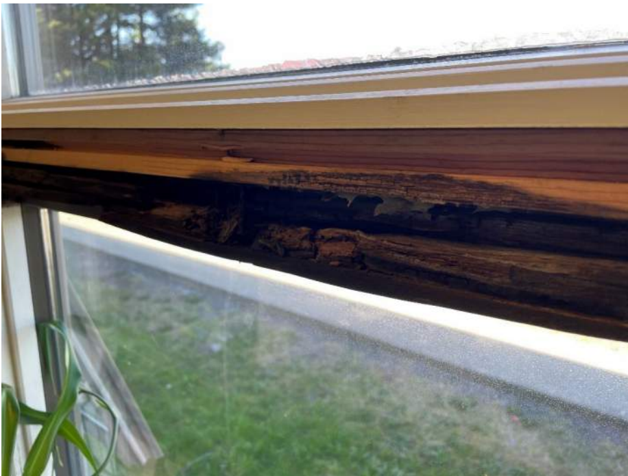
Rotting wood on north facing window units.
