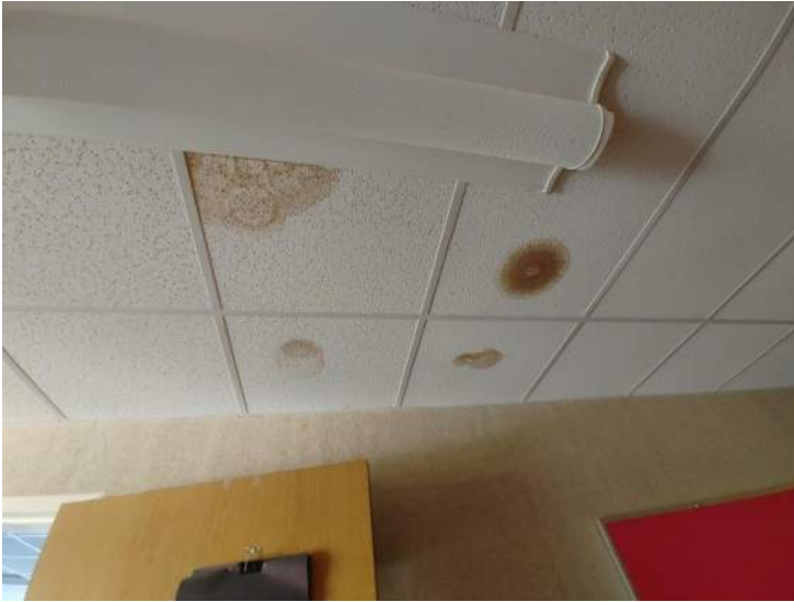
Water staining at ceiling tile, varies in hallways and classrooms
