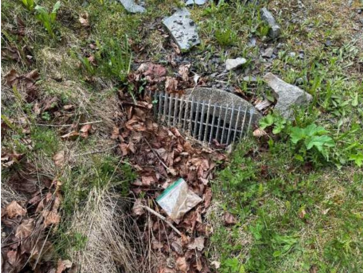
Inlet and pipe near east building corner
