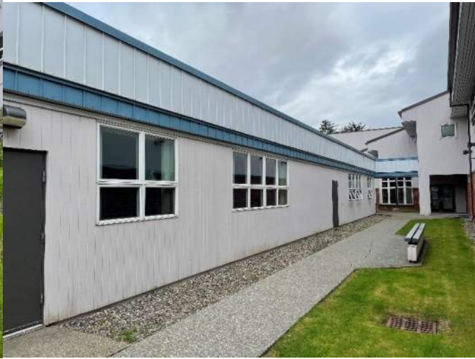
Upper level North side
