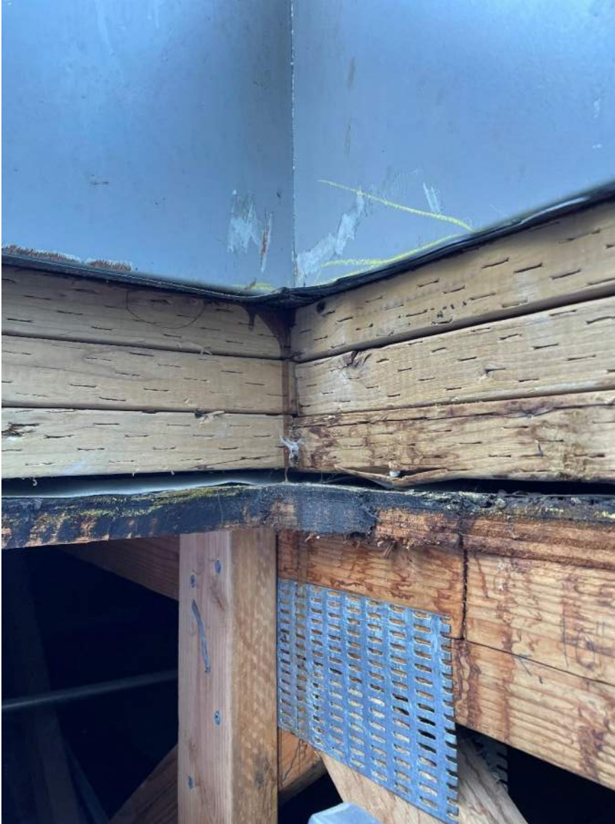
Roof assembly profile at access hatch curb.
