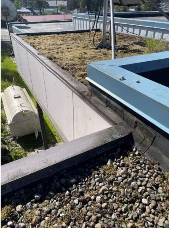
Ballasted north canopy roof
