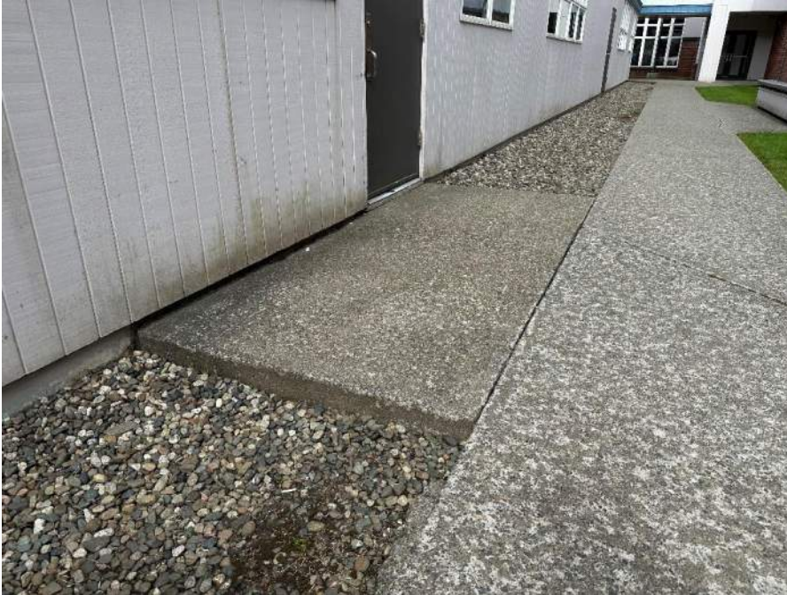
Replacing existing 10'x5' concrete stoop at door exiting building
