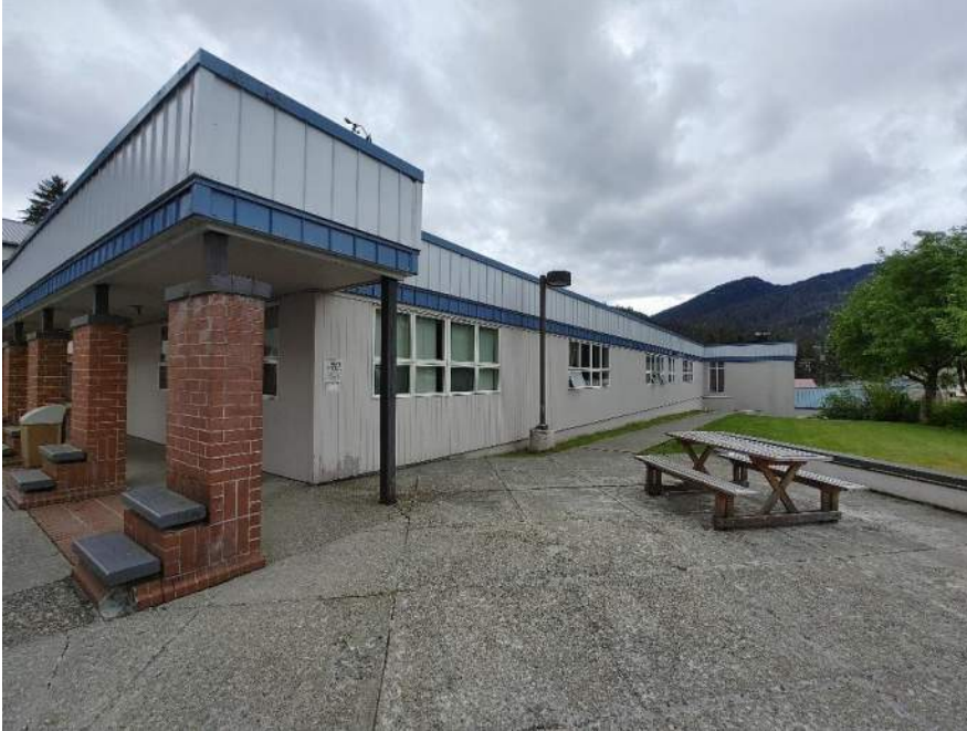
Picnic table and timber seat walls at upper patio, southwest corner.
