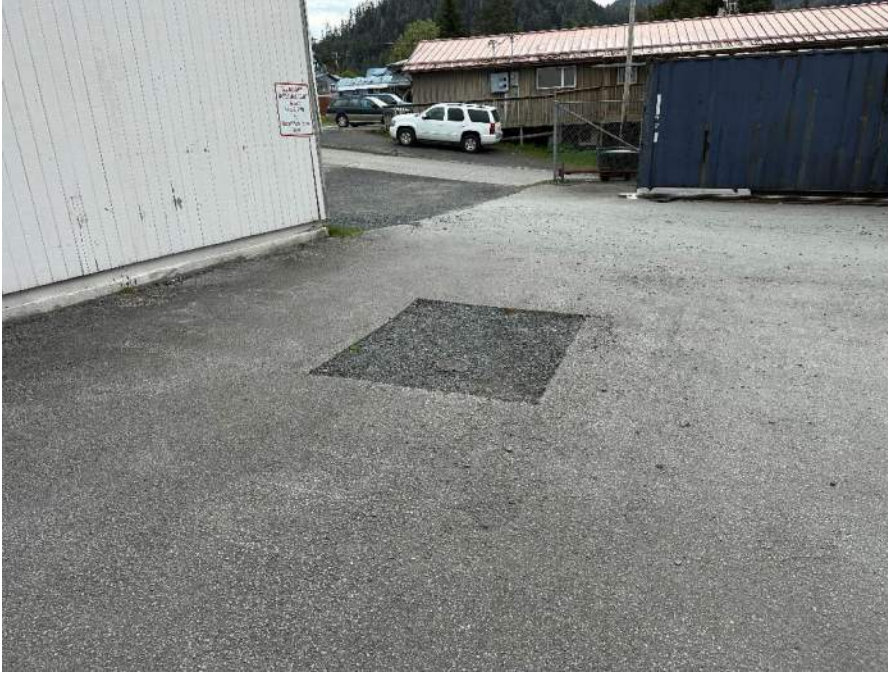
ACP cutouts around cleanouts
