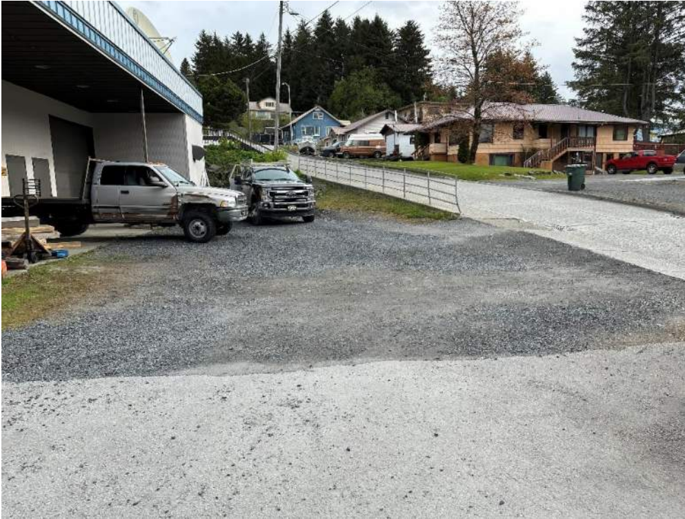
Re-grading vocational gravel parking area at southeast end of building.
