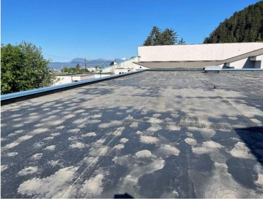
Looking west from Penthouse.
