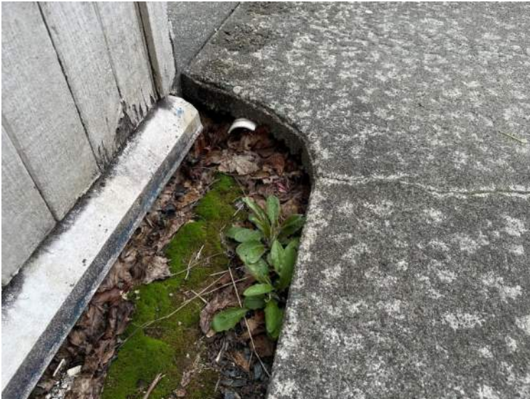
Drain pipe immediately northwest of building entrance on Church Street
