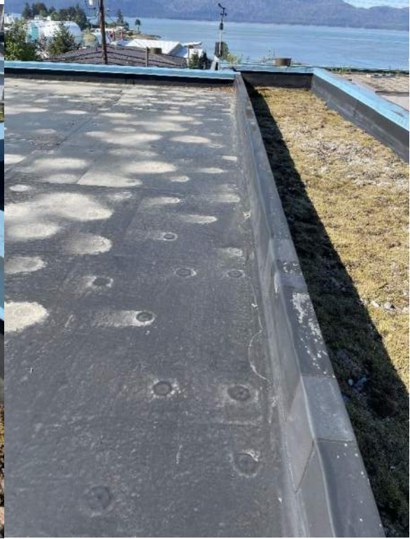
West Canopy roof meeting insulated building roof
