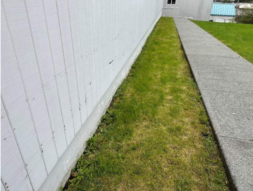
Vegetative buffer on northwest side of building, top level
