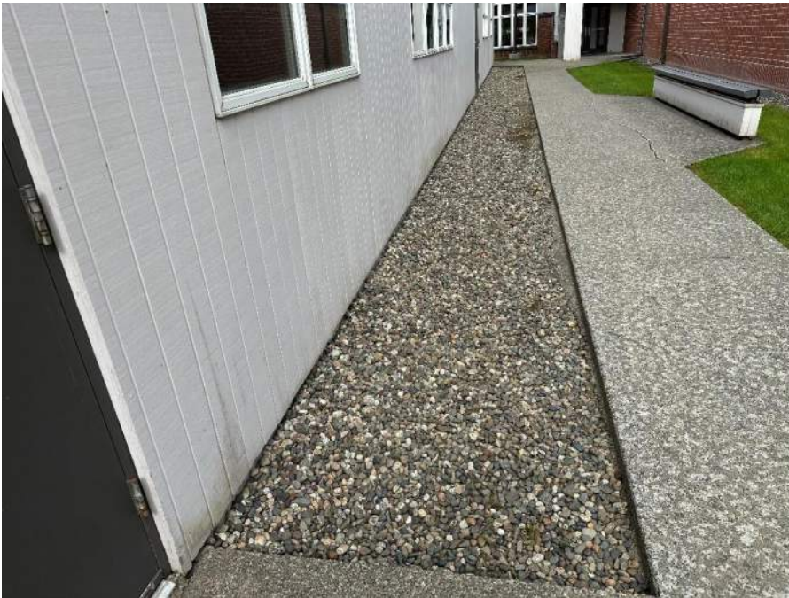
Buffer on northeast side of building, top level
