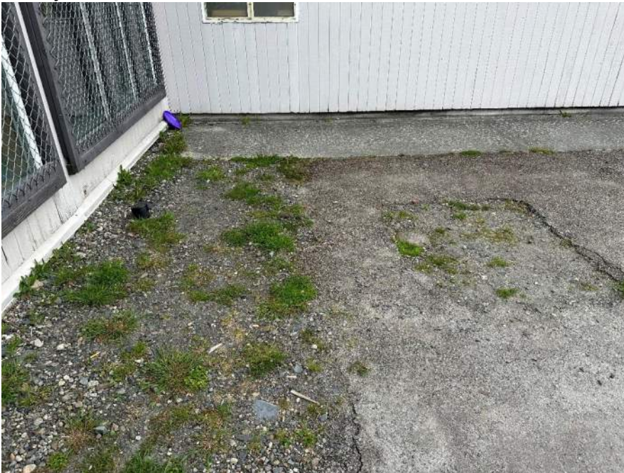
Remove weeds along building and pavement edges
