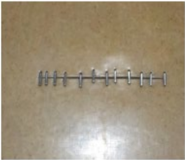
Deficiency Item S11. Example of existing vinyl flooring repair.
