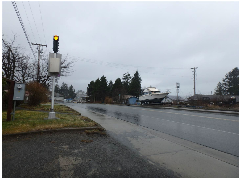
Bennett St viewing east
