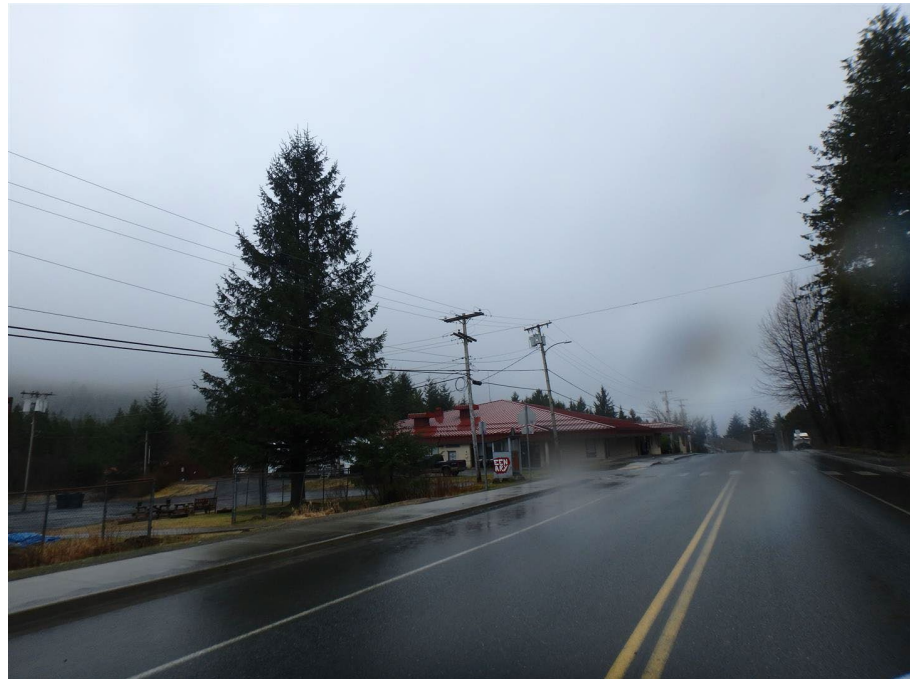
Bennett St viewing west
