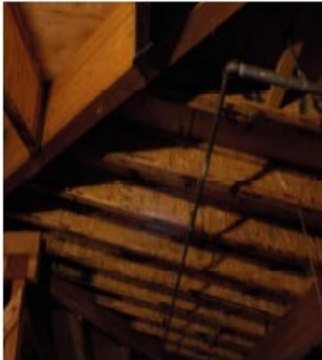
Typical structural roof framing in good condition. 1988 roof over-framing addition.
