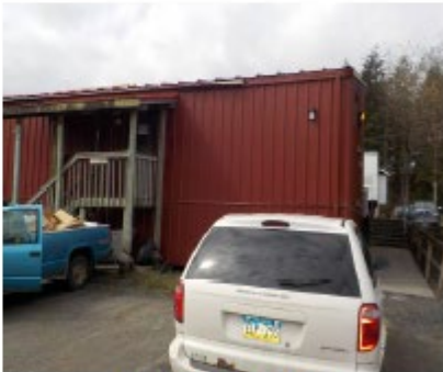
East Elevation - Shop 1994 Addition
