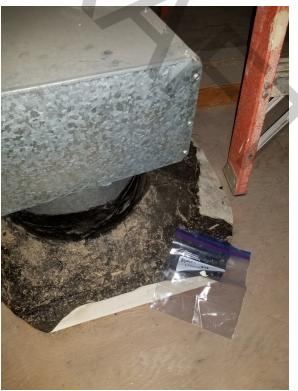
**Photo 2:** Tar paper skirts around penetrations in the new portion of the attic are ACM. (May 23, 2018)
