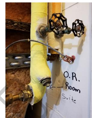
Photo 15: Exposed ends of presumed ACM TSI hard insulated joints. (May 22, 2018)
