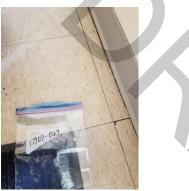
**Photo 6:** Off-white floor tiles in the stairway were ACM, and had a black mastic with trace amounts of asbestos. (May 22, 2018)
