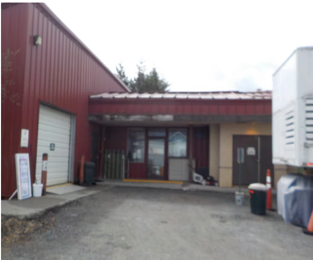
North Elevation – Shop Vestibule Shop to the Left 1994 Addition
