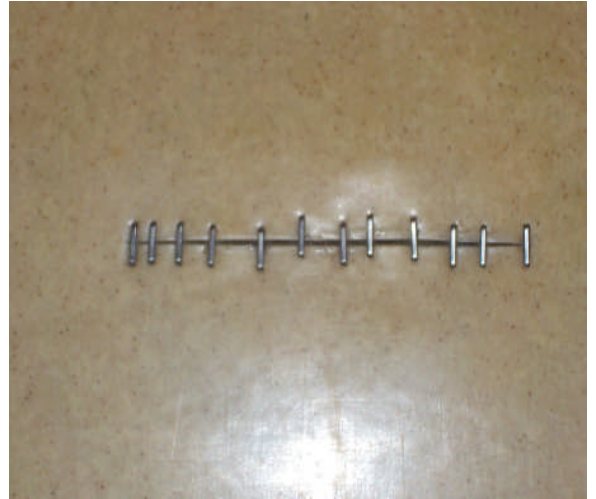
Deficiency Item S11. Example of existing vinyl flooring repair.
