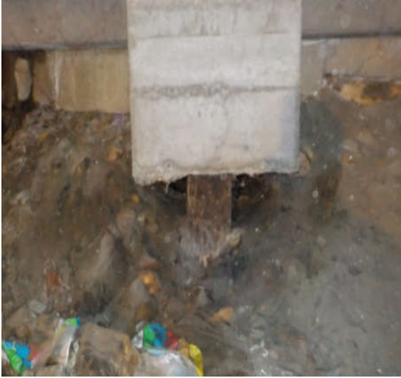
Typical creosote treated timber piling beneath 1968 Construction, beneath kitchen. In good condition. Reinforced concrete pile cap and grade beams in good condition.
