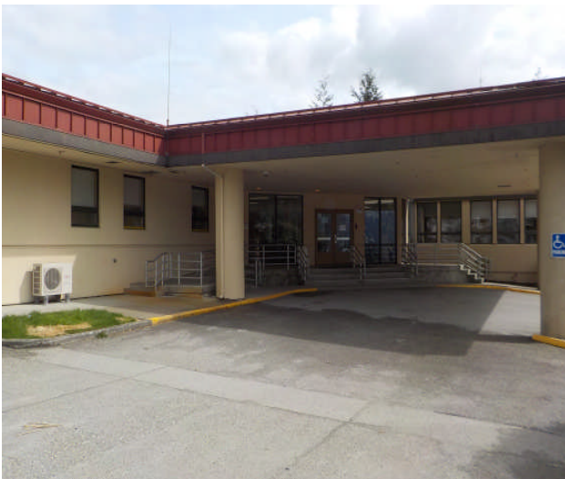
Main Entry – Southwest Elevation
