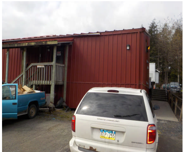
East Elevation - Shop 1994 Addition
