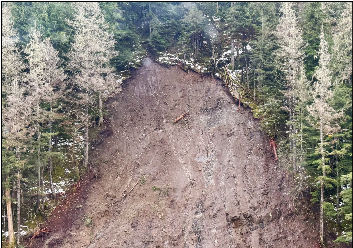
Figure 12. MP11.2 landslide head scarp (photo by Barrett Salisbury, November 23, 2023).
