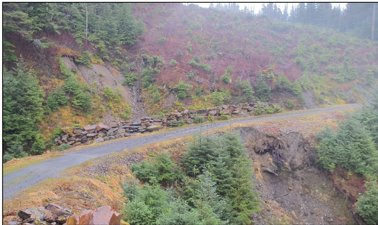
Figure 8. Existing landslide on forestry road 50052 (photo by Jillian Nicolazzo, November 25, 2023).
