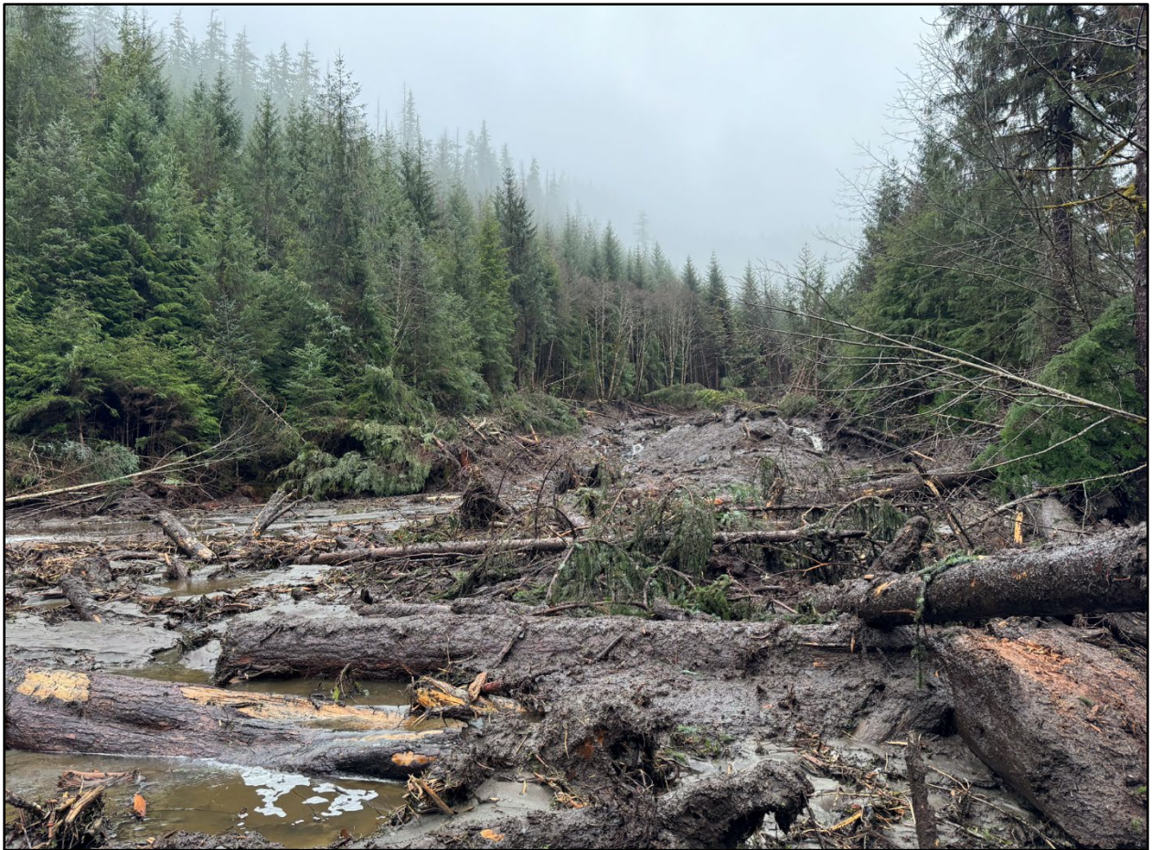
Figure 6. Toe of the Middle Ridge Road landslide where it covers the road (photo looking south by Barrett Salisbury, November 24, 2023).
