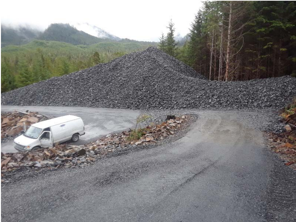
Photo 3: Stockpiled rock at Monofill Site
