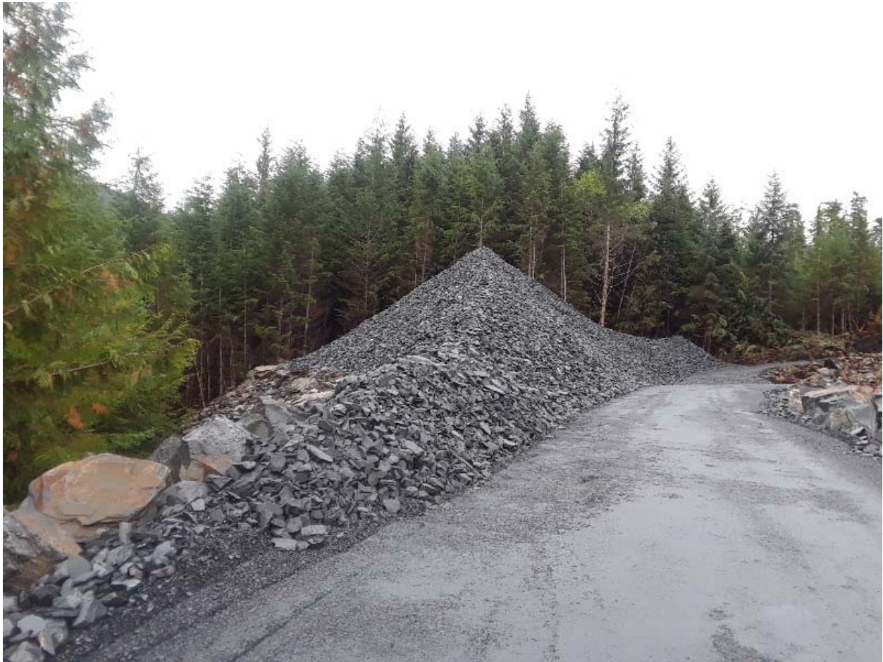
Photo 2: Stockpiled rock at Monofill Site
