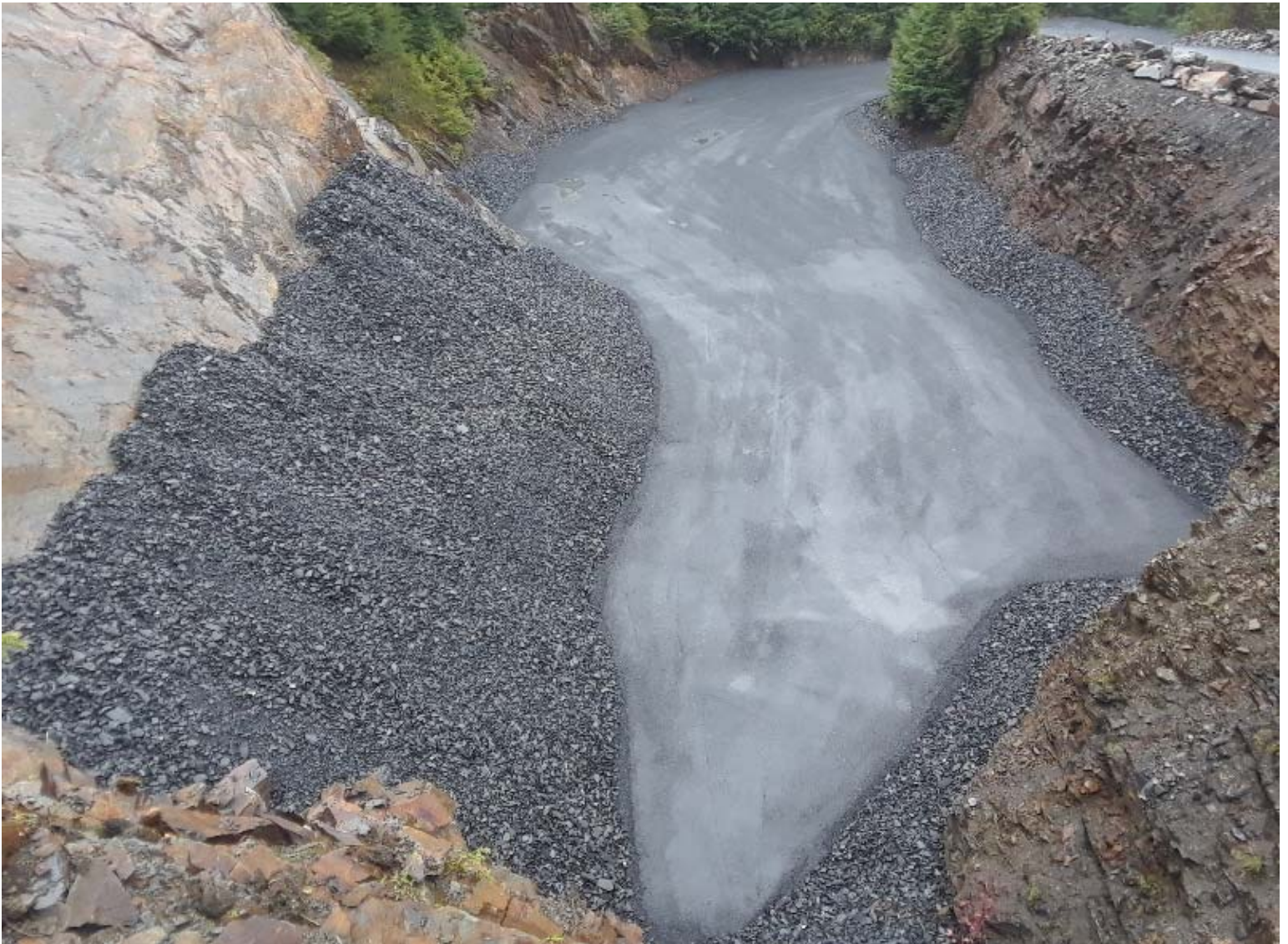
Photo 1: Monofill Site, Base Drain complete, start of Chimney Drain
