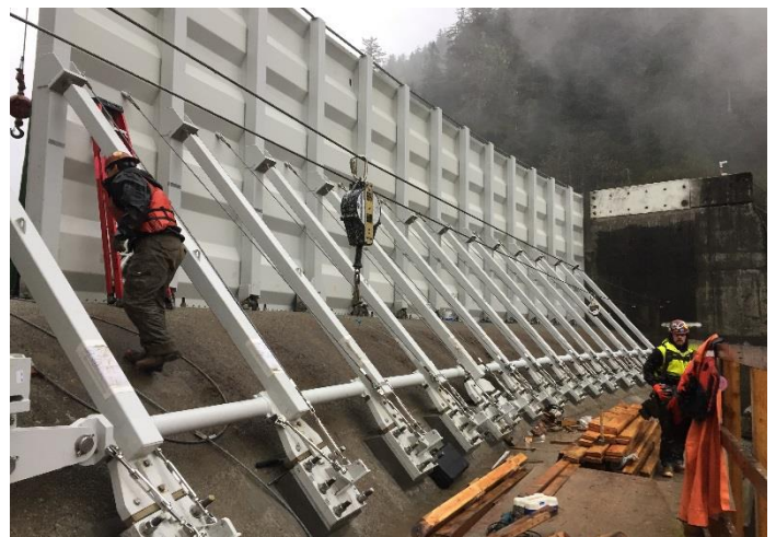
Placing flashboard panels between columns
