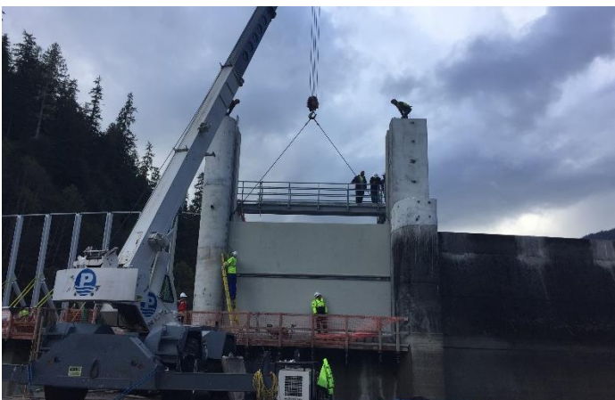
Top half of vertical gate lowered into place
