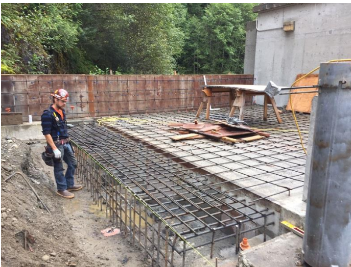
Intake building watertight parapet wall and bulkhead
