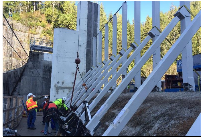
Installing flashboard kicker assemblies
