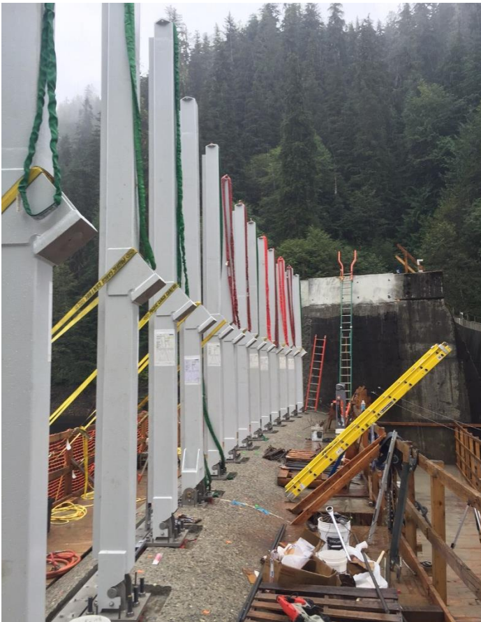
Flashboard columns erected
