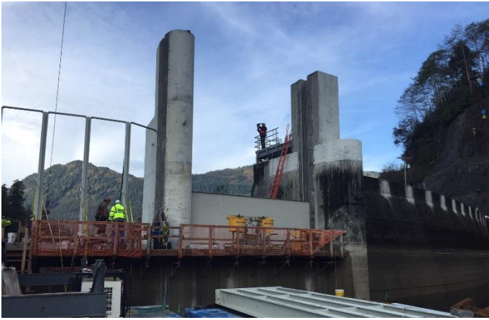
Lower half of vertical gate in place
