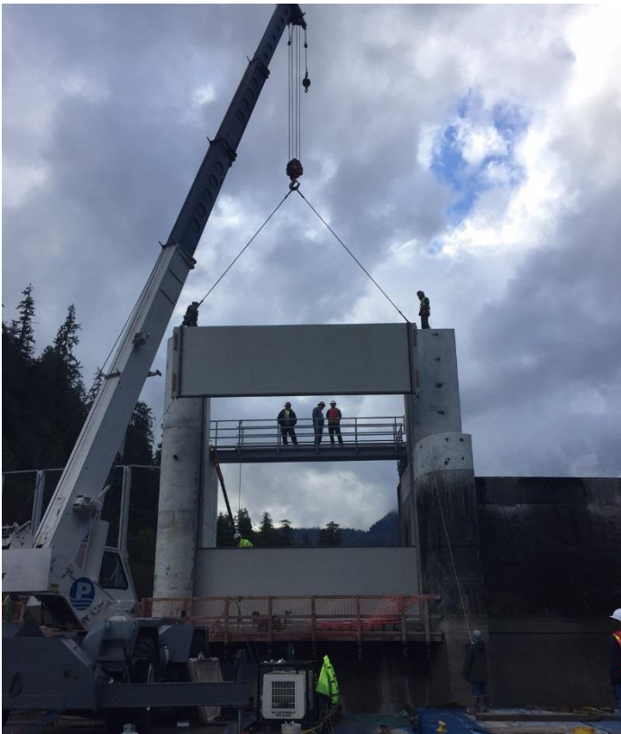
Lifting upper half of vertical gate into slot
