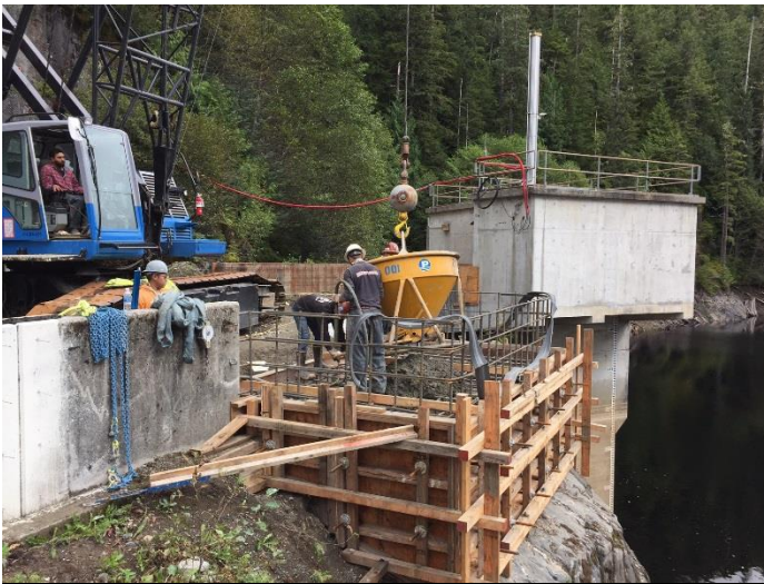
Placing log removal platform concrete
