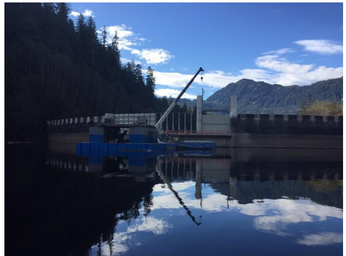
Perspective view of spillway work
