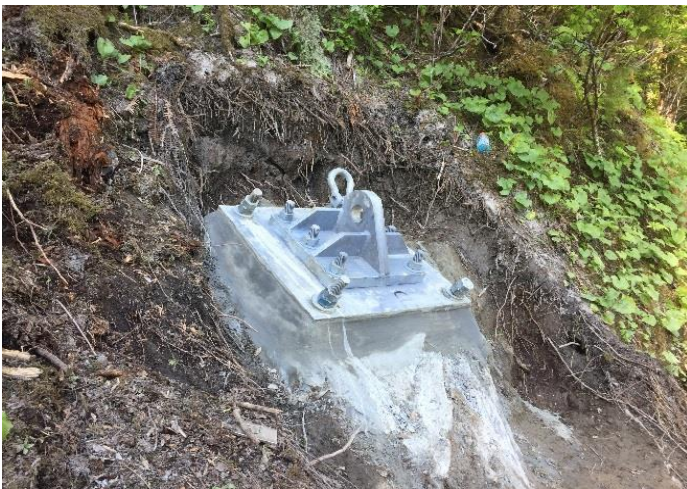
New Debris Boom Shore Anchor (Complete)
