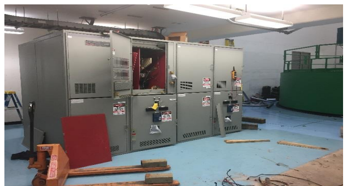
Unit 1 New Switchgear Cabin Installed
