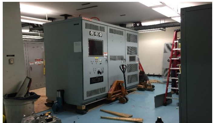
Removing Unit 1 Exciter Cabinet
