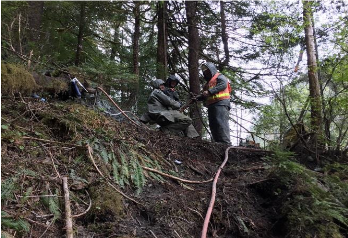
Hand Drilling Shore Anchors
