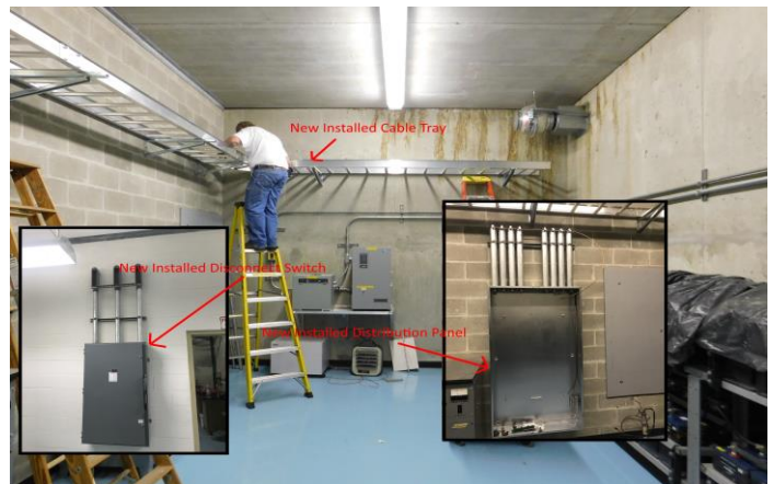
Installation of a new 125VDC Distribution System at Swan Lake will create redundancy, increase reliability and enable standard maintenance to be performed without requiring a powerhouse outage.
