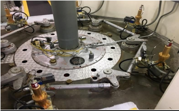
All twelve (6 per turbine) needle restoring mechanism position feedback assemblies were replaced with an improved design that will enhance reliability and serviceability (brass colored).
