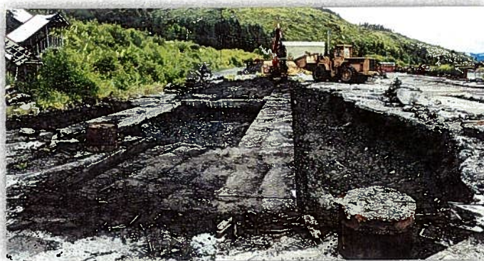
Figure 6: Looking south along the former green chain line area on 6/29/12. Excavations exposed 4'-wide foundations which later were discovered to be the former hydraulic-powered 'action pack'
