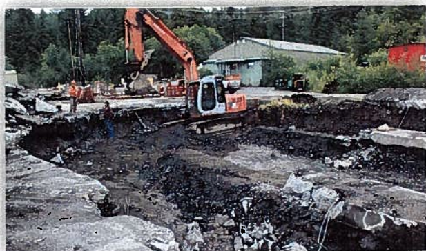
Figure 7: View on 7/20/12- looking toward the north end of the green chain/ sorter line after the former 'action pack' foundation had been removed for continued excavation of contaminated soil
