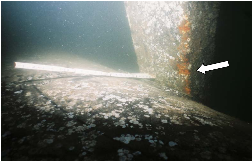
PHOTO No. 9: Seven Foot Diameter Floatation Tank – Note the good condition of the welded connection between the square tubular strut and the floatation tank. Also not the good condition of the epoxy coating on the top of the pontoon and the localized coating failure on the strut.
