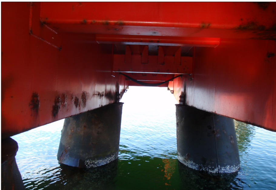
Ramp/support tank connection assembly.
