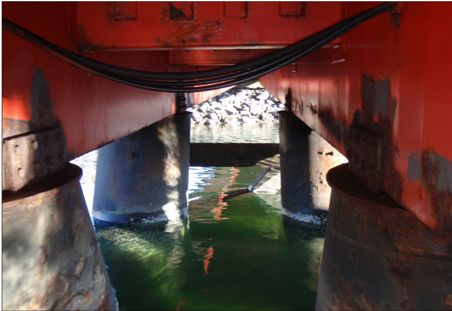
Ramp/support tank connection assembly.
