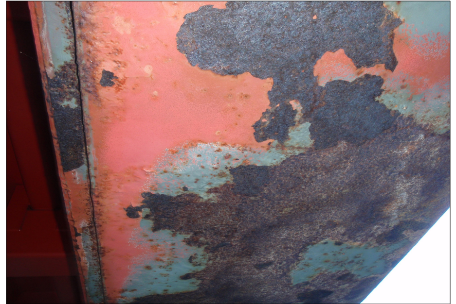
Typical coating failure/corrosion of girder bottom flange.
