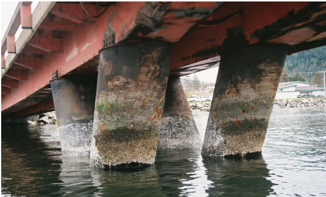
PHOTO No. 4: Floatation Tank Pipe Struts – Note the deterioration and failure of the protective black epoxy coating on these members in the splash zone.
