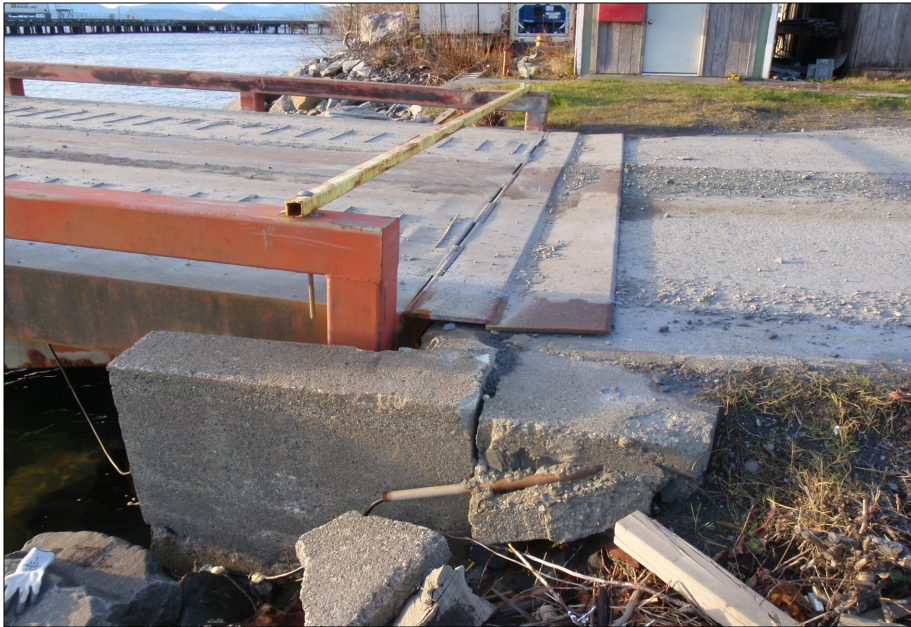
Transition plate at barge ramp abutment.
