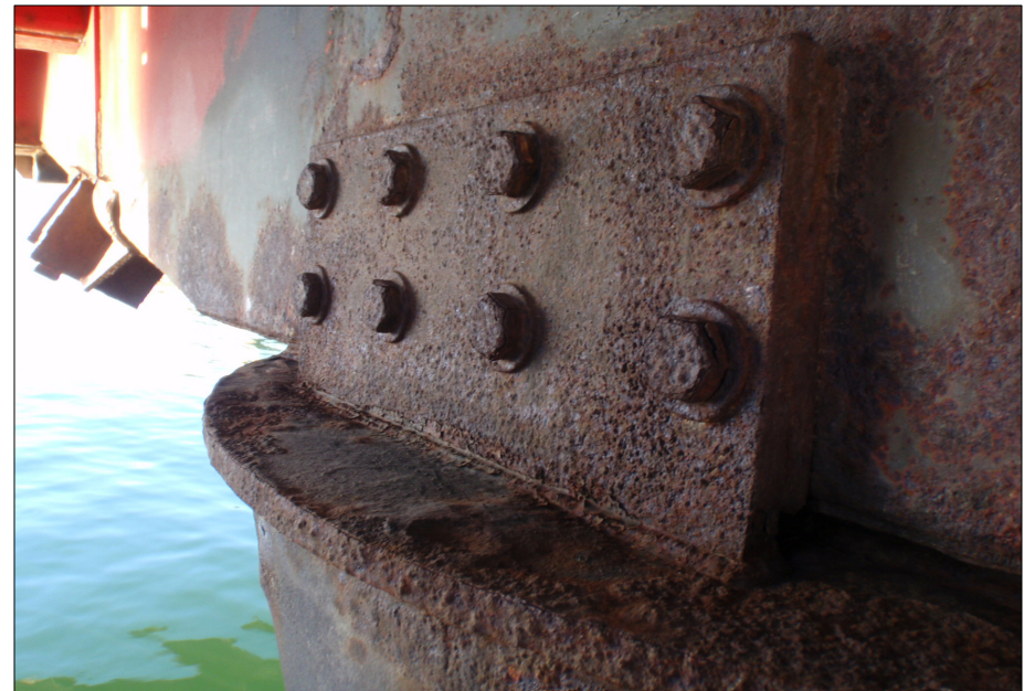
Coating failure/corrosion at ramp/support tank connection assemblies.
