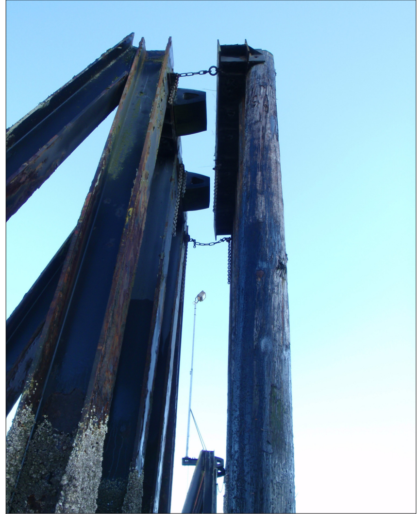
Broken stay chains at Dolphin "C".
