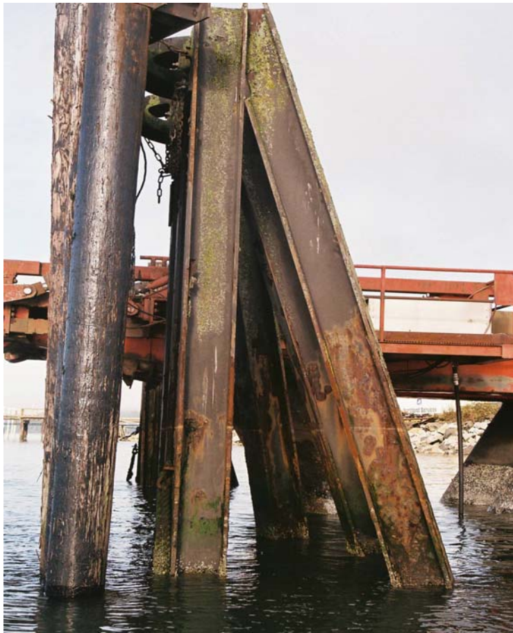
PHOTO No. 11: Breasting Dolphin F – Note the good condition of the epoxy coating at the tops of the piles and the localized coating deterioration in the splash zone. Overall these piles have been estimated to retain 75% of their coating in the combined top and splash zone.
