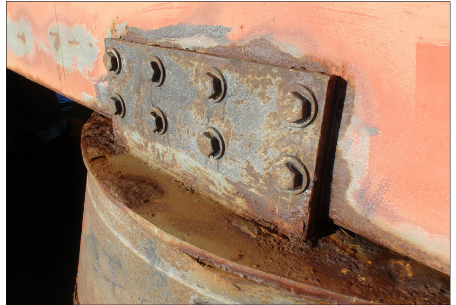
Coating failure/corrosion at ramp/support tank connection assemblies.
