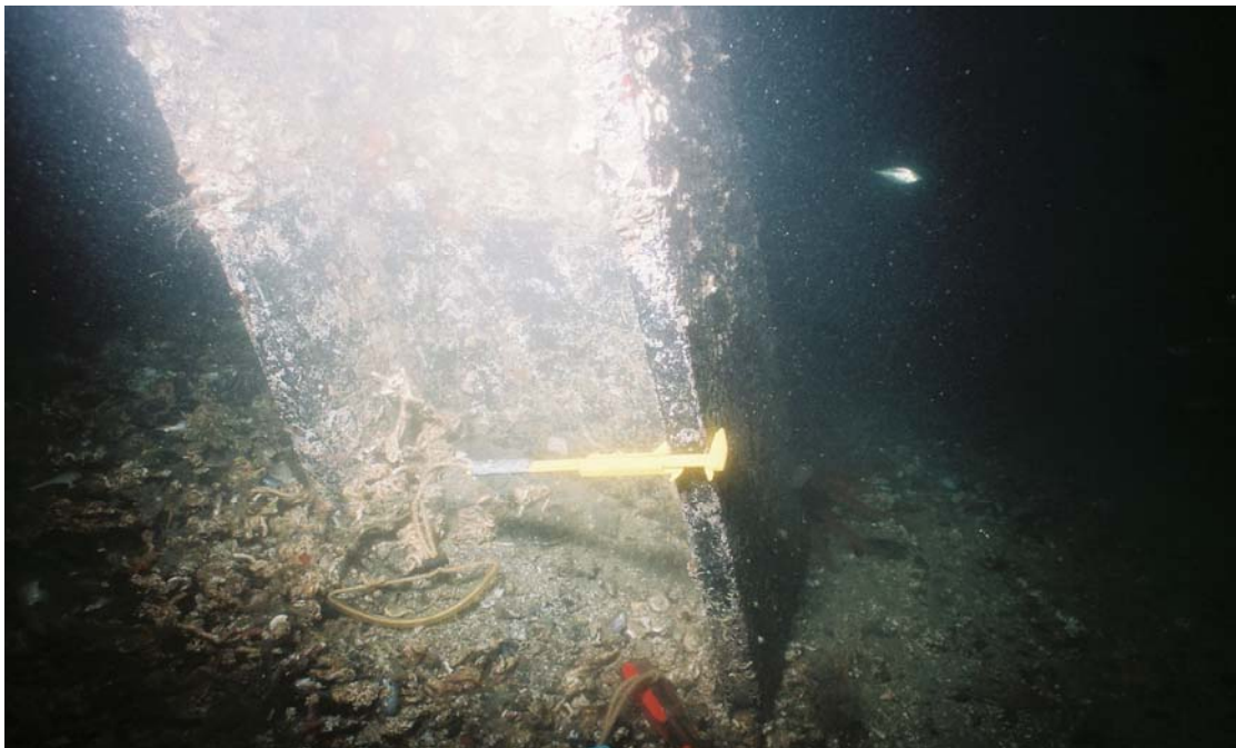
PHOTO No. 14: Breasting Dolphin C, Pile 3 Batter – Level II cleaning of this pile at the mudline found it to be in good condition with an estimated 90% of the epoxy coating intact at the mudline.
