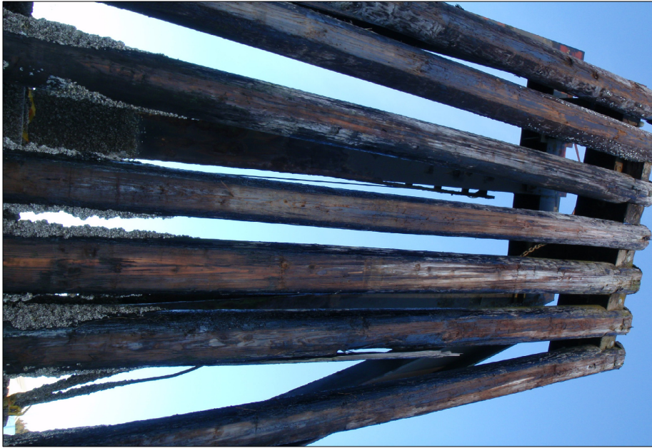
Displaced fender piles at Dolphin "D".
