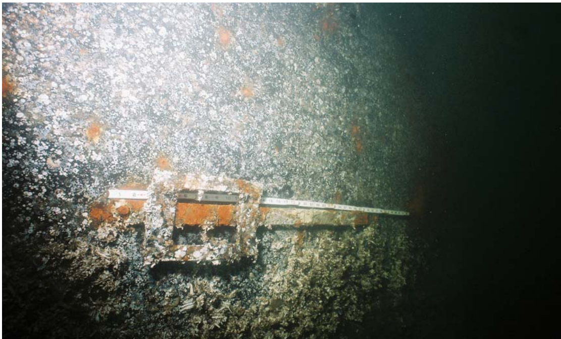
PHOTO No. 6: Floatation Pontoon Cathodic Protection Anode Bracket – Investigation of the Floatation Tanks noted this anode bracket on the north end of the larger 9 ft. diameter tank. Note the ruler lying along the top of the anode attachment bracket. The anode has been completely consumed.
