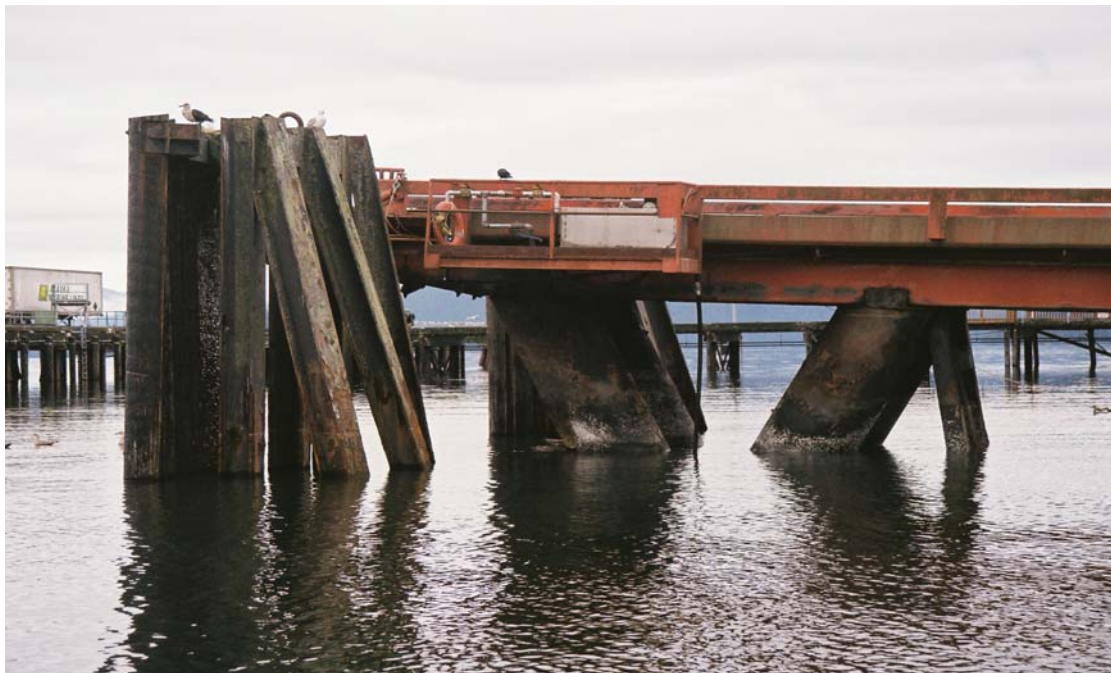
PHOTO No. 2: Barge Facility Transfer Span – Note the large diameter pipe struts that connect to a nine foot diameter floatation tank located ~3 feet below the surface. The square tube struts shoreward of the pipe struts connect to a second smaller pontoon (7 foot diameter). Also note Dolphin F in the foreground.
