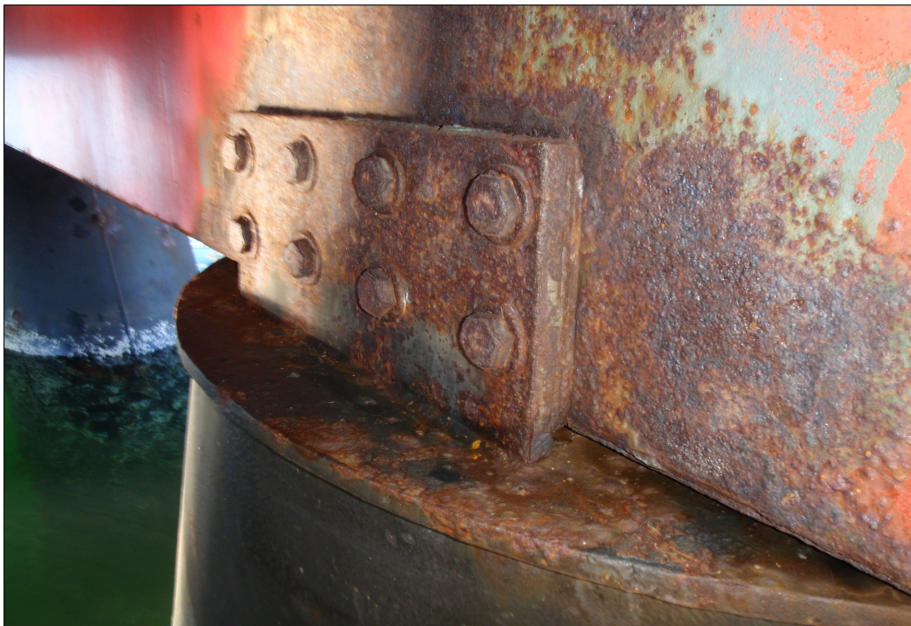
Coating failure/corrosion at ramp/support tank connection assemblies.
