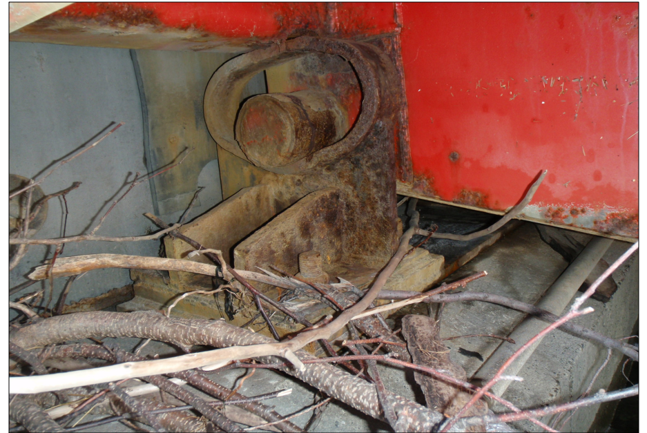
North bearing assembly, debris and worn steel; coating failure on all steel components.
