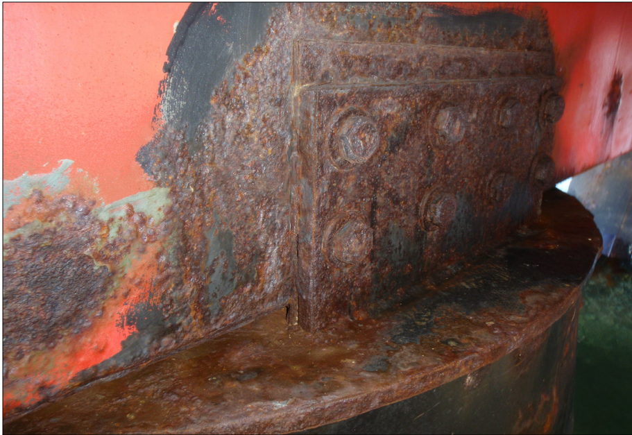
Coating failure/corrosion at ramp/support tank connection assemblies.
