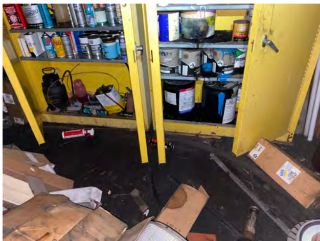
Photo 22: Looking at containers inside the flammable storage cabinets, located in the mezzanine of the main shop structure.
