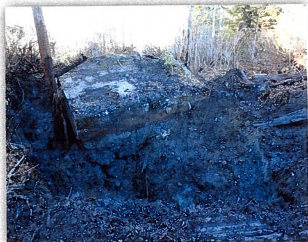
Figure 12: The 10/26/12 view of the city-tie transformer site excavation
