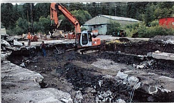
Figure 7: View on 7/20/12- looking toward the north end of the green chain/ sorter line after the former 'action pack' foundation had been removed for continued excavation of contaminated soil
