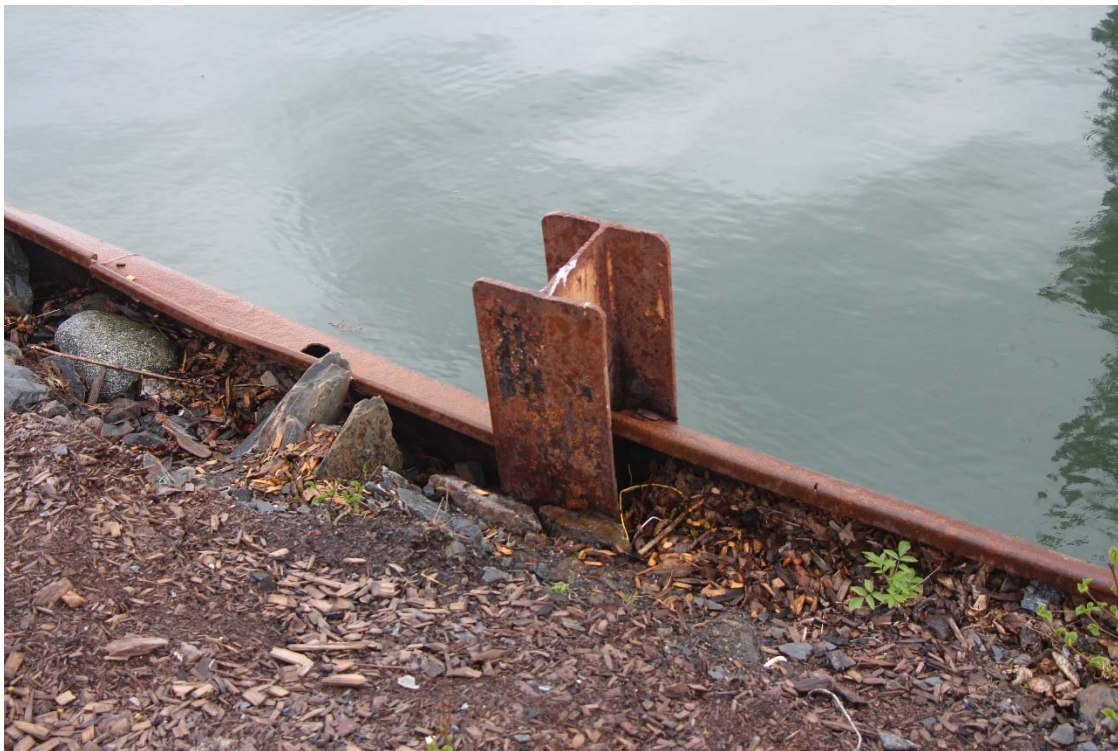
Photo 7 – H-Pile at Railroad Car Bulkhead
