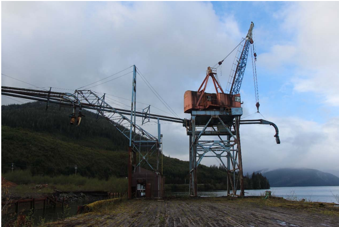
Photo 5 –Tower Crane and Conveyor Support
