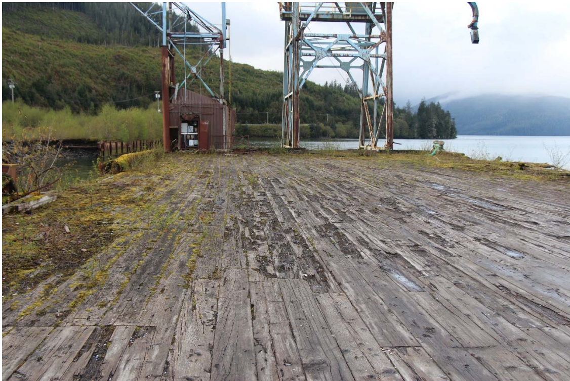
Photo 3 – Timber Pier Deck (looking south)
