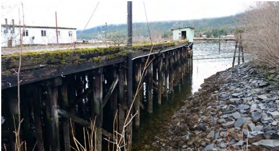
Photograph 2. Condition of the pier.
