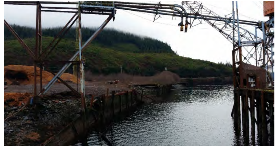
Photograph 3. Condition of the bulkhead adjacent to the pier.
