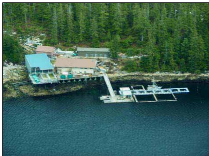
SSRAA Burnett Hatchery
