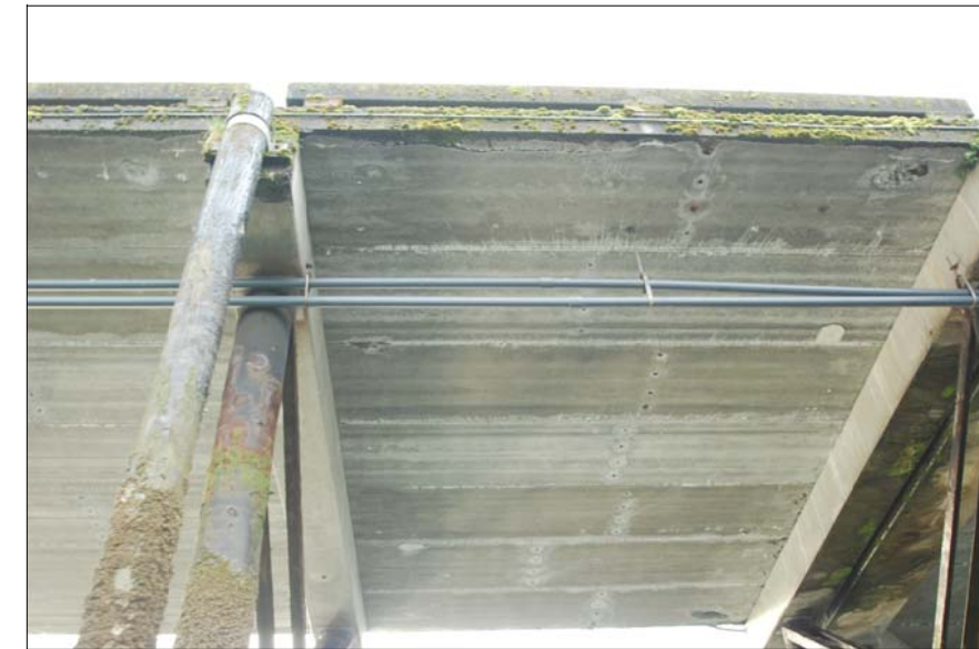
(A) EXISTING WATERLINE HANGERS - PHOTO
