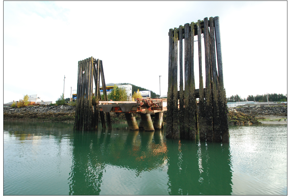
Barge ramp, looking north.
