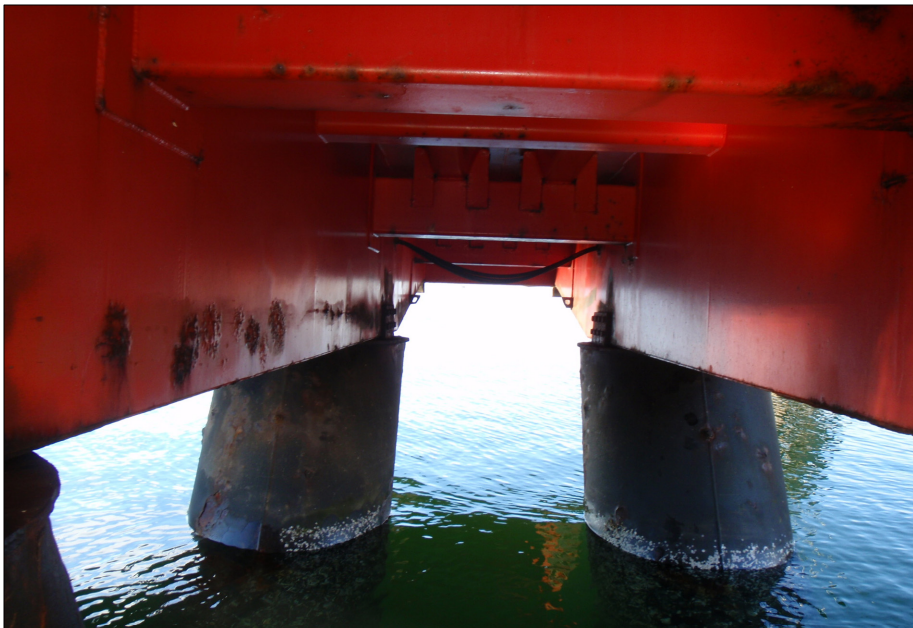
Ramp/support tank connection assembly.
