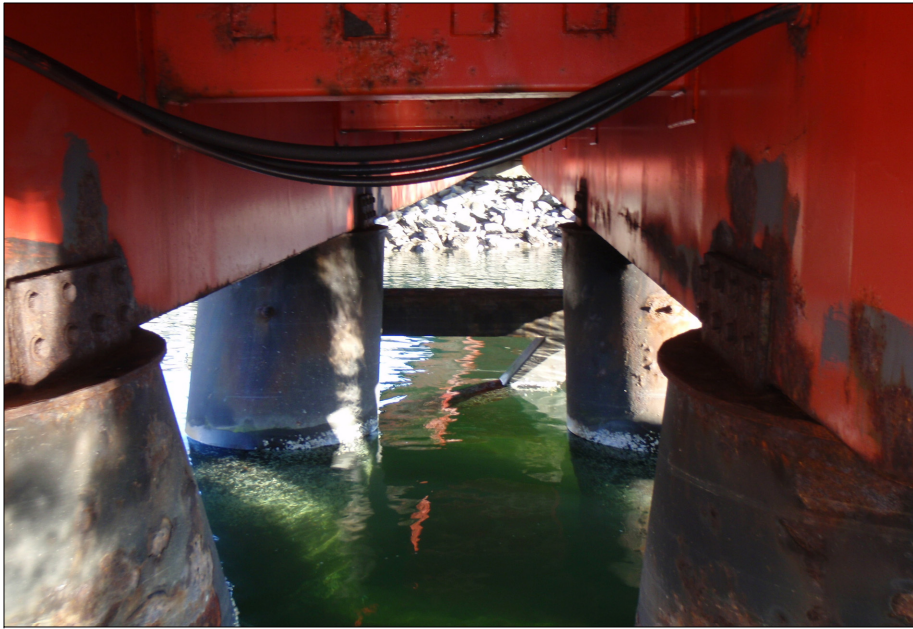
Ramp/support tank connection assembly.
