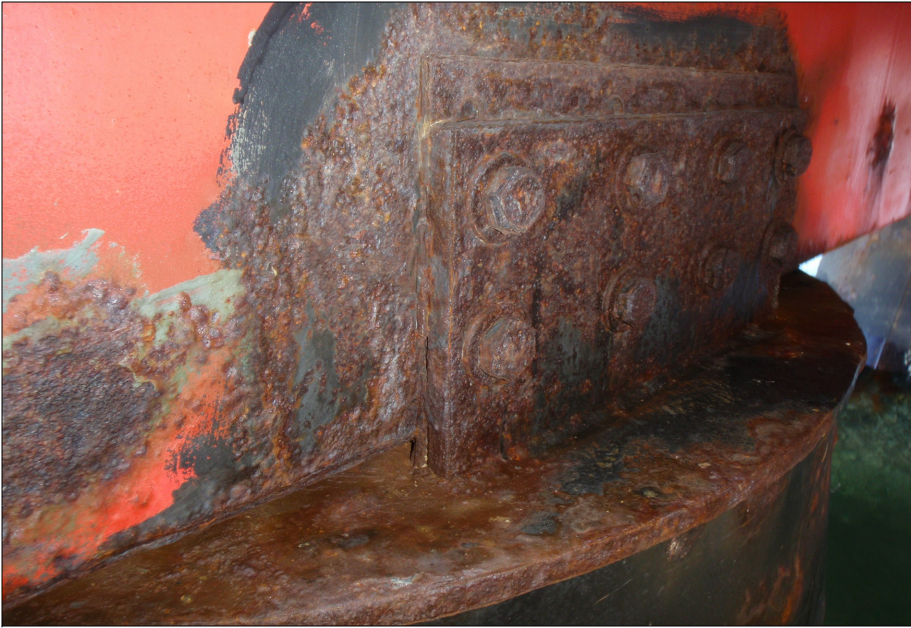
Coating failure/corrosion at ramp/support tank connection assemblies.
