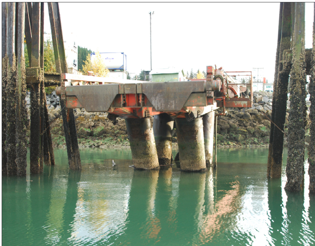
End of barge ramp, looking shoreward.
