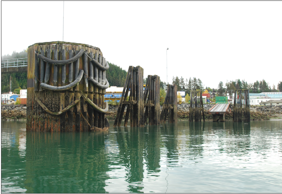
Overall view of barge ramp facility, looking east.
