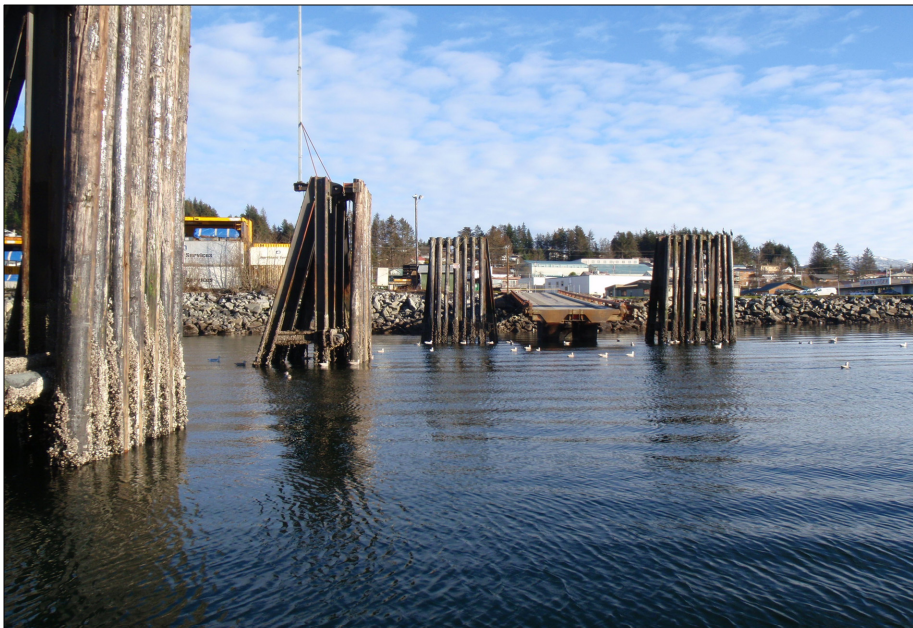
Barge ramp, looking east.
