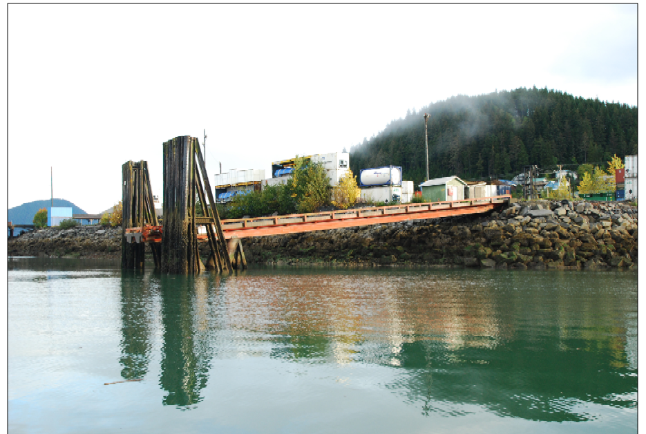
Overall barge ramp, looking north.
