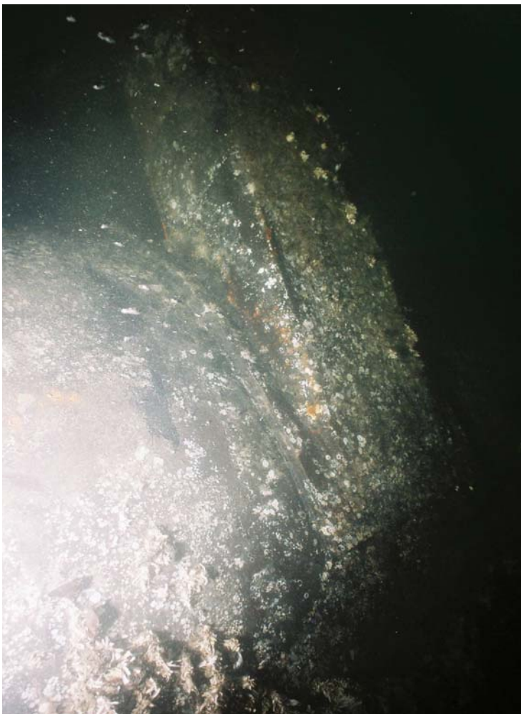
PHOTO No. 10: Seven Foot Diameter Floatation Tank – Note the good condition of the welded connection between the square tubular strut and the eastern side of the floatation tank. Also note the general good condition of the epoxy coating.
