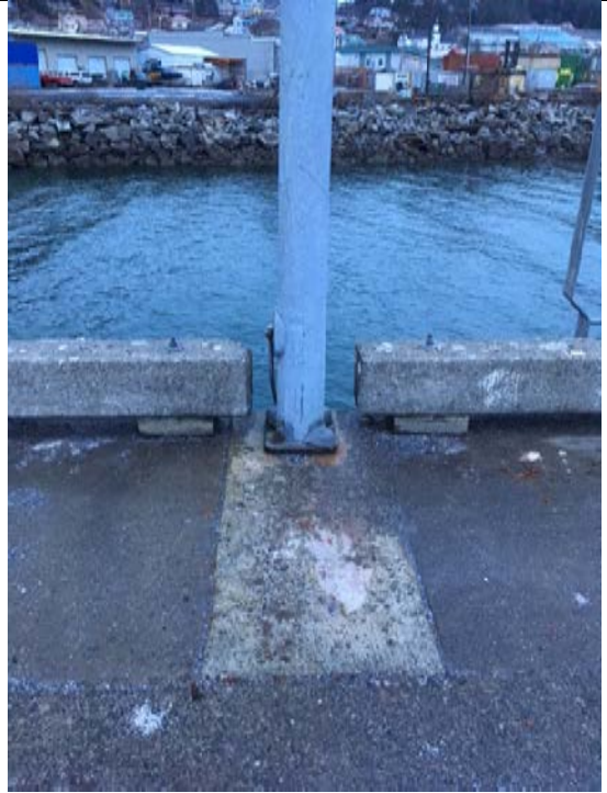
Light Pole Base on Main Dock Lower South End
