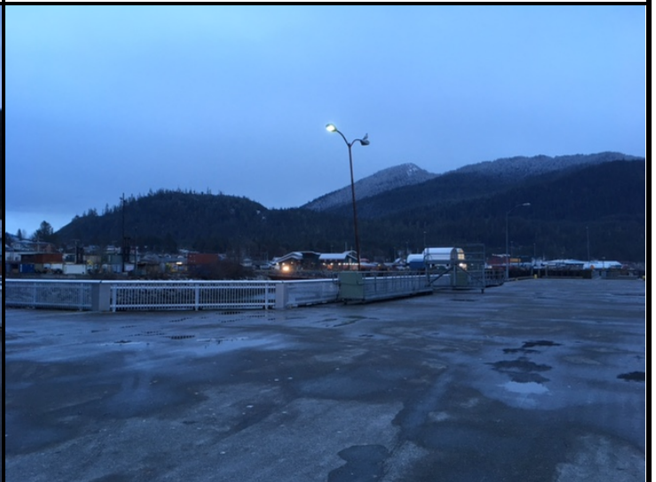
View of Main Dock North End
