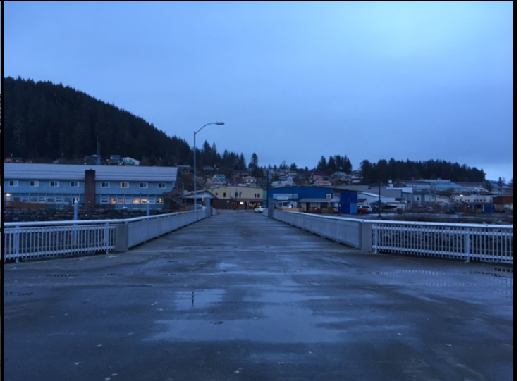
View of Approach Dock from Main Dock
