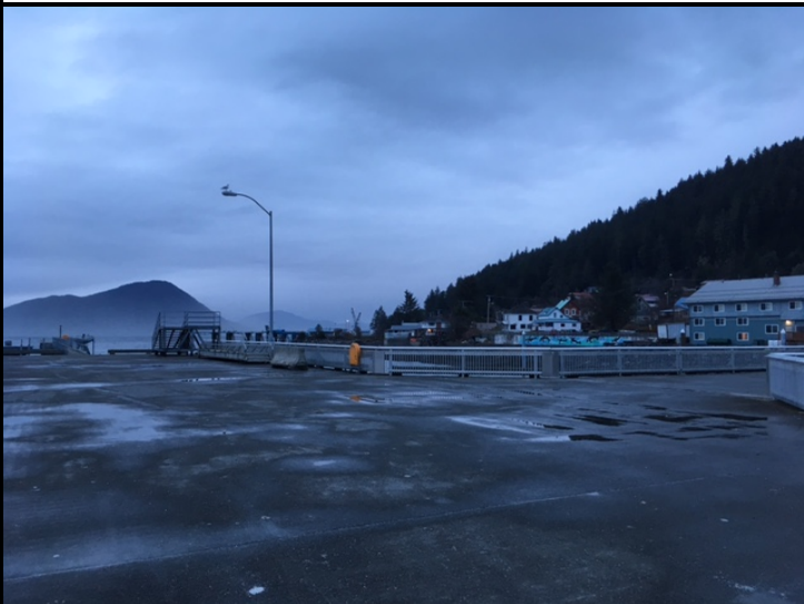
View of Main Dock North End
