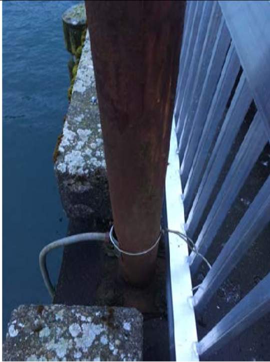
Light Pole Base on Main Dock Upper South End
