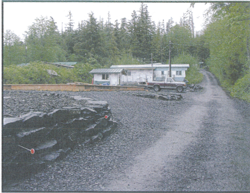
Figure 10 - View looking up at area vulnerable to inundation
