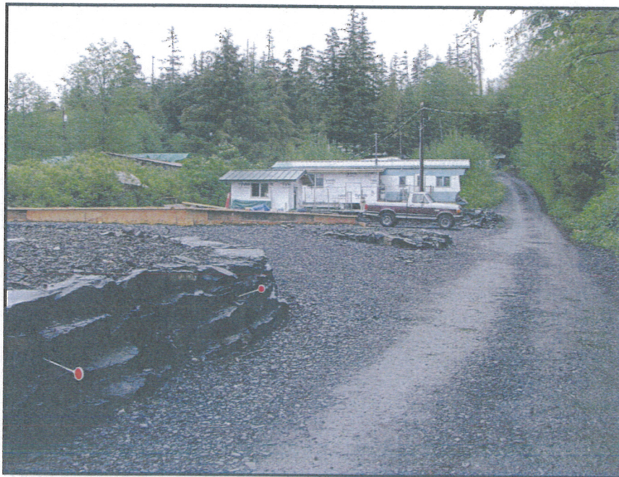
Figure 6 - View looking up at area vulnerable to inundation
