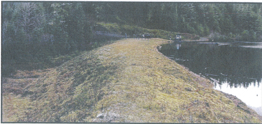
Figure 8. Wrangell Upper Dam
