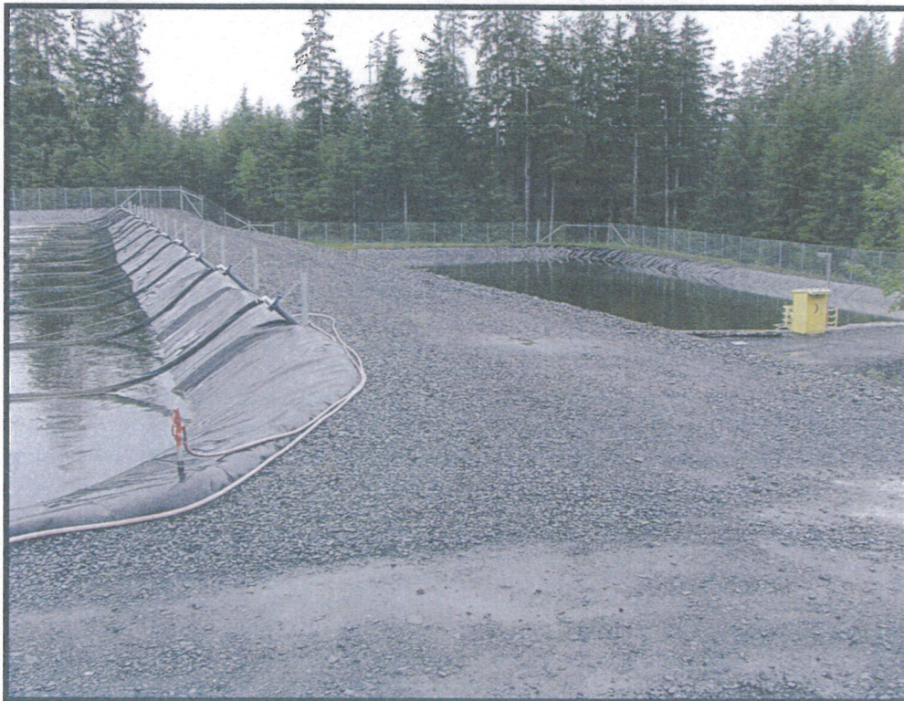
Figure 11 - City of Wrangell sewage treatment plant
