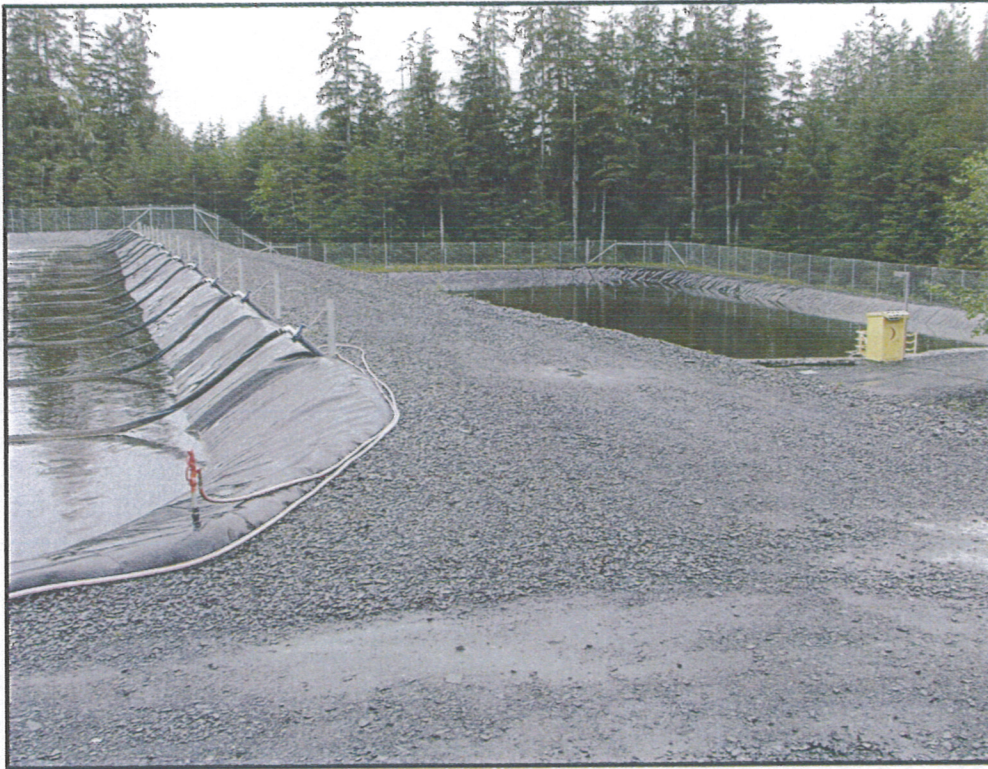
Figure 7 - City of Wrangell sewage treatment plant
