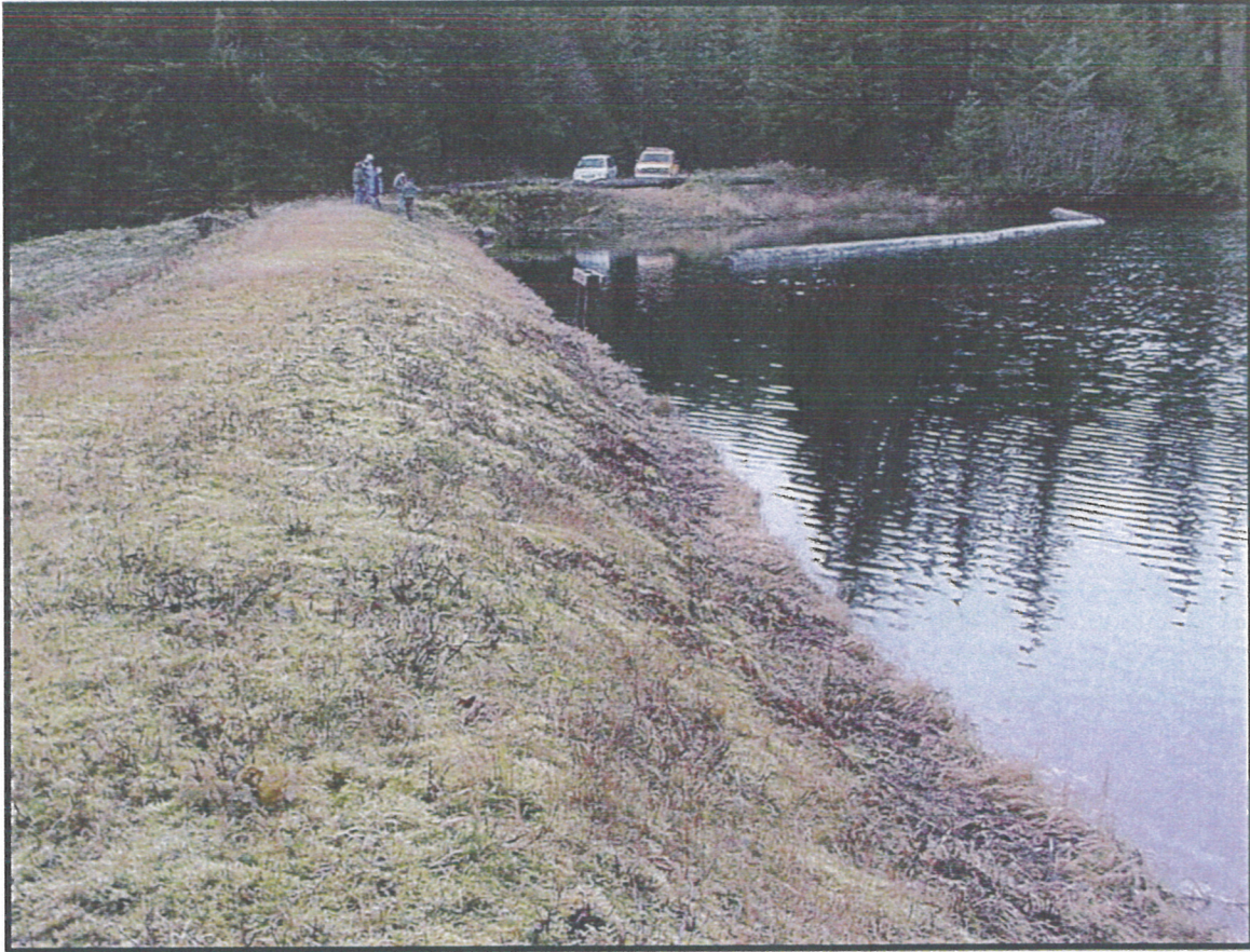
Figure 9. Wrangell Lower Dam
